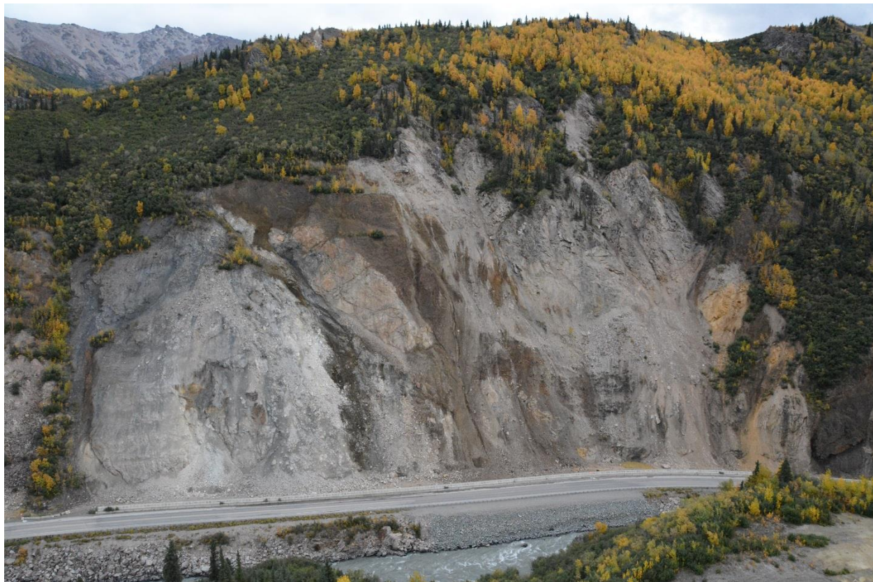
Figure 12: MLS scanning on the Parks Highway, Alaska with an aerial oblique photo from an alternate vantage point. Note the MLS data is limited to the approximately bottom third to half of this very tall slope.
