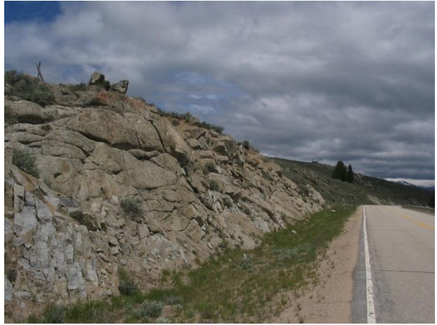
'Good' Condition Slopes exhibiting stability and an effective ditch.
