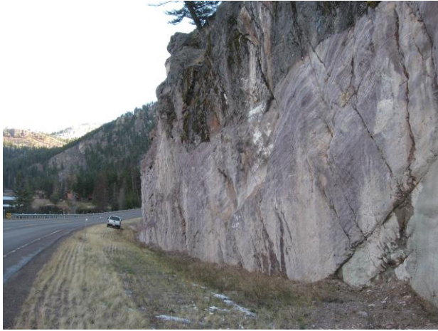
'Good' Condition Slopes exhibiting stability and an effective ditch.
