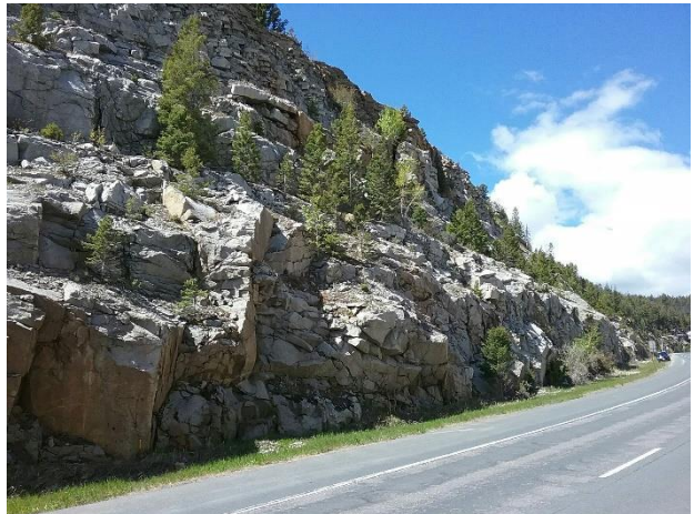
'Fair' Condition Slopes with smaller, less effective ditches and with more rockfall activity.
