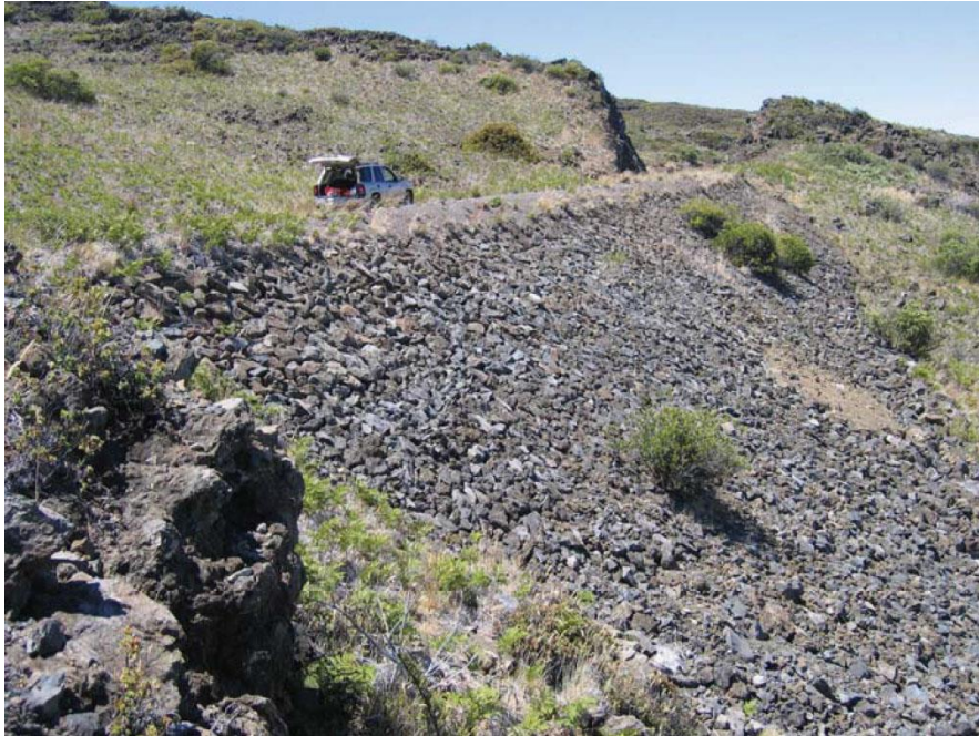
Figure 2: Geotechnical feature with ambiguous classification
