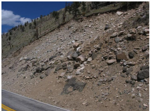
'Poor' Condition Slopes exhibiting high levels of activity and ineffective ditches.
