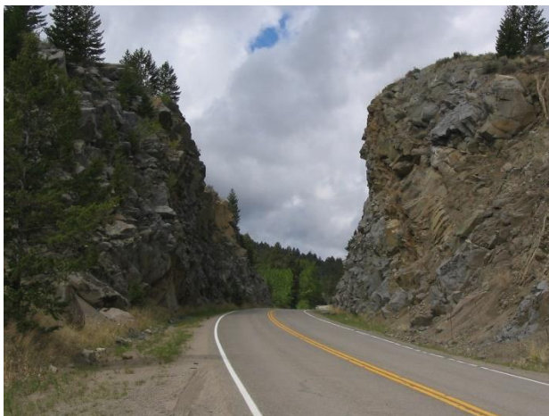
'Poor' Condition Slopes exhibiting high levels of activity and ineffective ditches.
