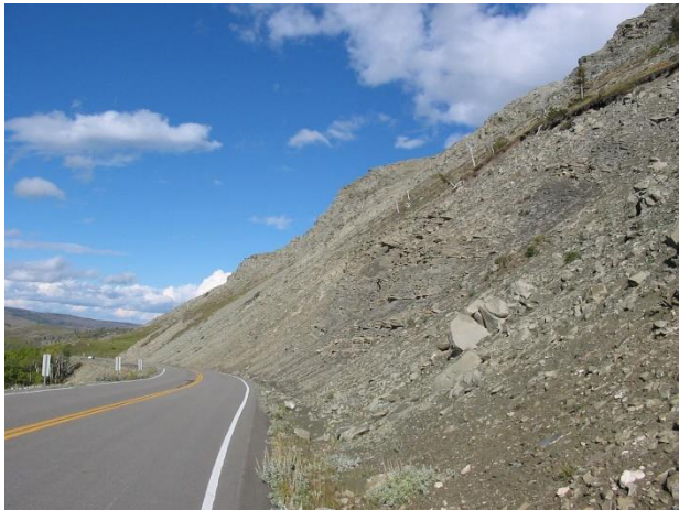
'Fair' Condition Slopes with smaller, less effective ditches and with more rockfall activity.
