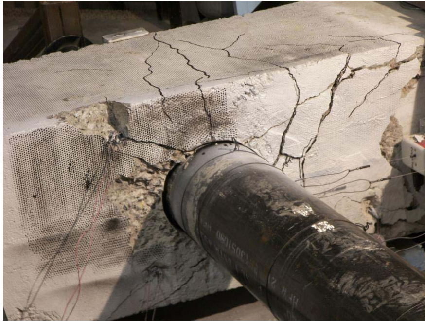
Figure 42: VT2.5 Failure at maximum negative deflection
