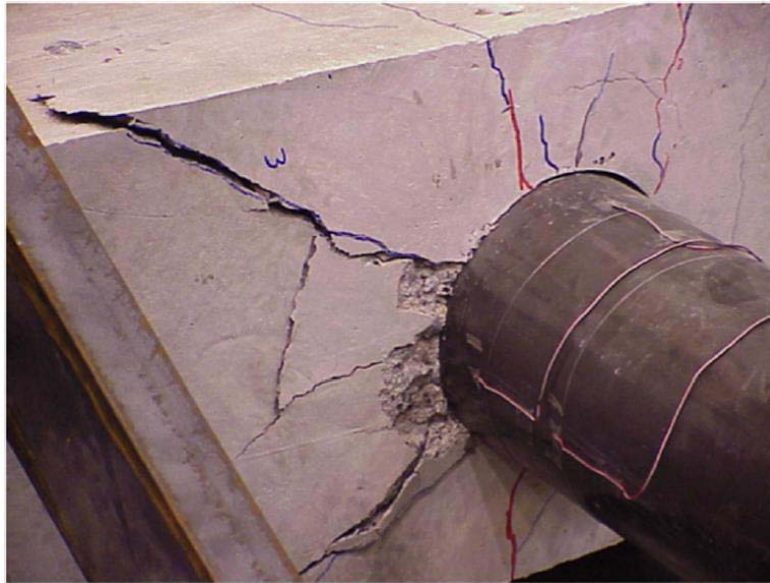
Figure 11. Typical failure mechanism observed in Phase I effort
