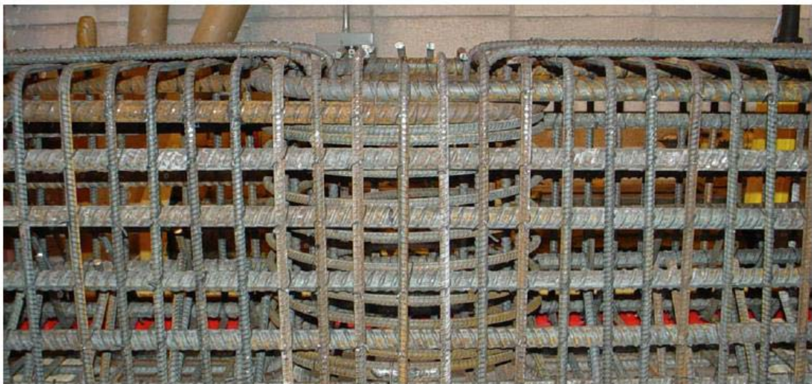
Figure 12. Reinforcing cage from Phase I PC4
