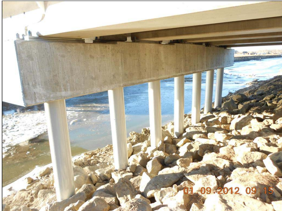
Figure 9. Typical bridge bent
