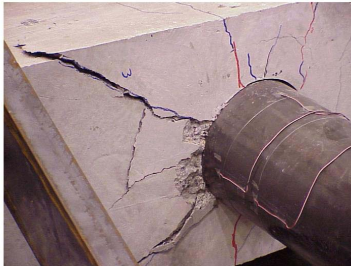
Figure 8: Typical Failure Mechanism seen in PC-1 through PC-3a (Stephens and McKittrick 2005)
