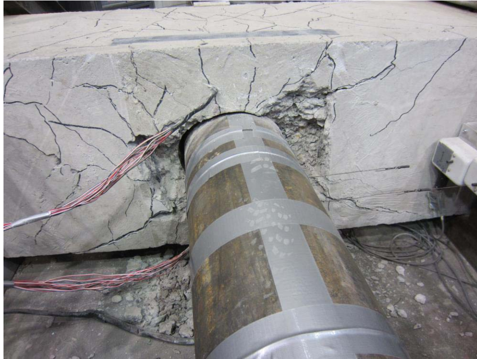
Figure 49: CT1 near the completion of testing
