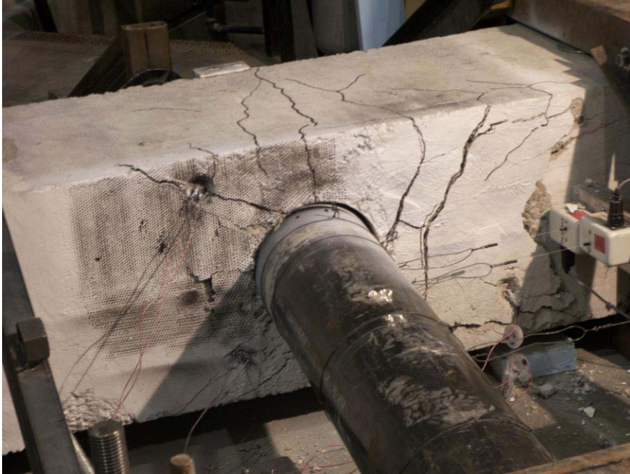
Figure 41: VT2.5 Failure at maximum positive deflection
