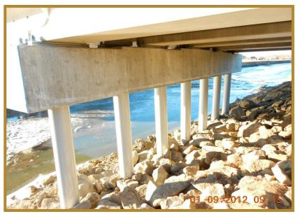
Figure 1 - Typical MDT Concrete-filled Steel Pipe and Concrete Pile Cap Bridge Substructure Support System
