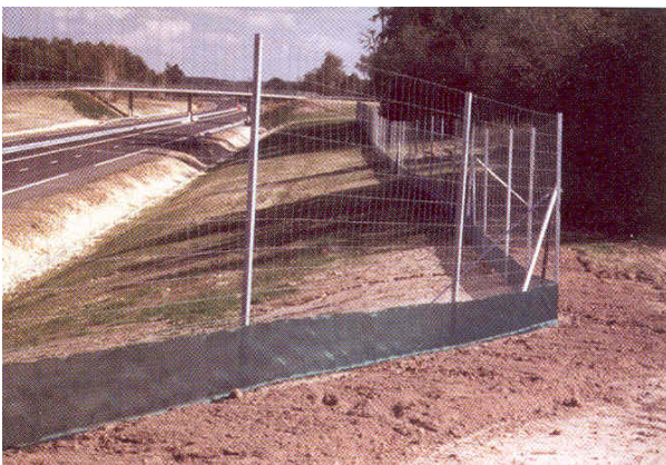
Figure A-1. Wire fence with plastic fabric mesh (France). Photo: Bank et al. 2002.
