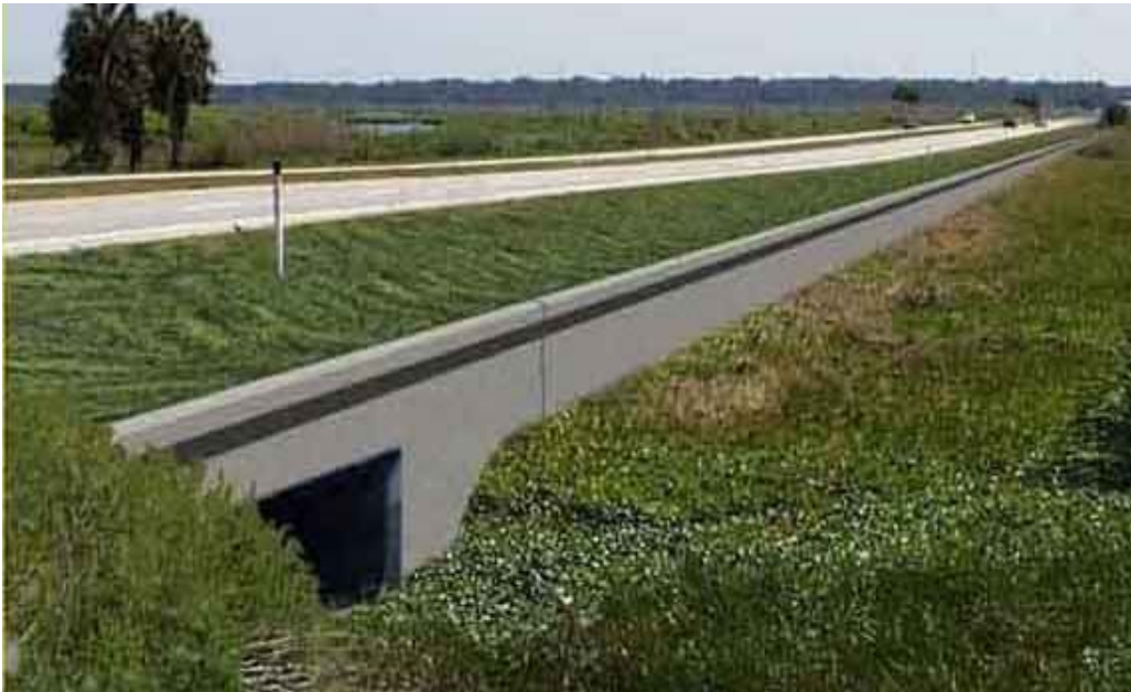
Figure A-7. Paynes Prairie Ecopassage (Florida) – Artist rendition. Concrete wall with lip. Photo: D. Forsyth. www.fhwa.dot.gov/environment/wildlifecrossings/amphibian.htm
