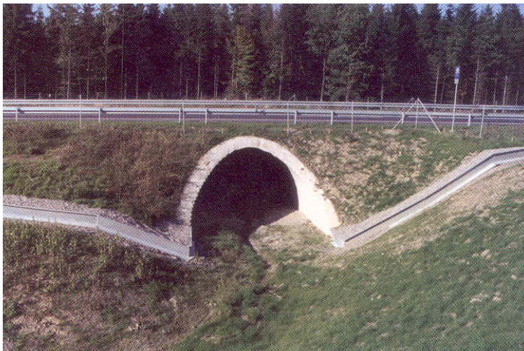
Figure A-12. Example of a combination of barrier methods. Arched culvert with large fence along highway and metal rail for amphibians and reptiles (Germany). Photo: Bank et al. 2002.
