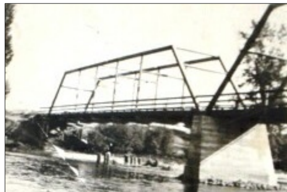
Figure 5-2. 1930s photo of the ca. 1920 bridge spanning the Bitterroot River.
