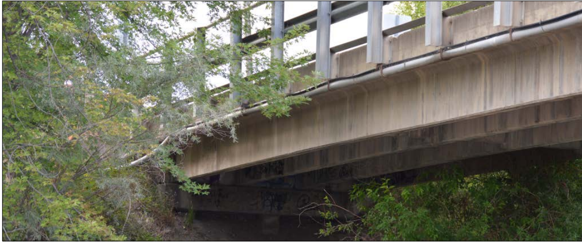
Figure 5-8. Prestressed concrete segment of Maclay Bridge.
