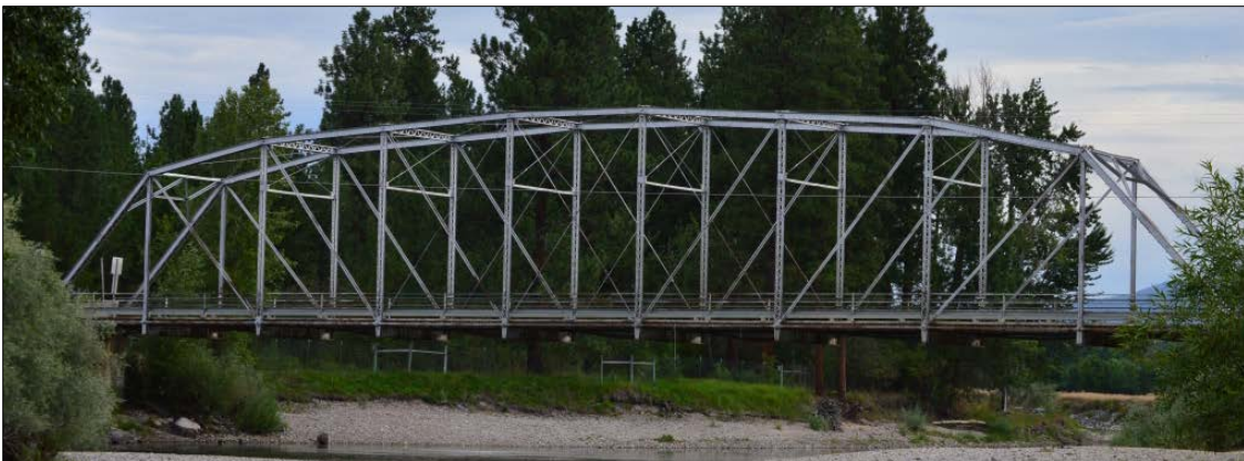
Figure 5-6. Parker truss segment of the Maclay Bridge.
