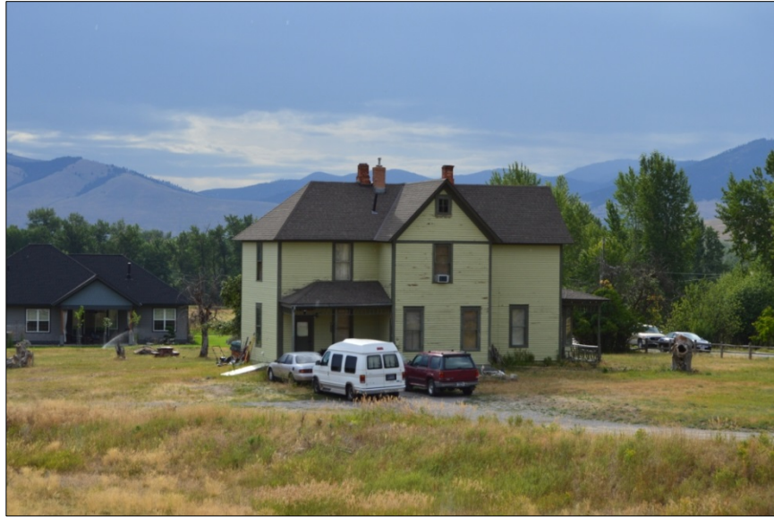
Figure 4-3. 24MO0519, the Maclay House, west elevation, view to the east.
