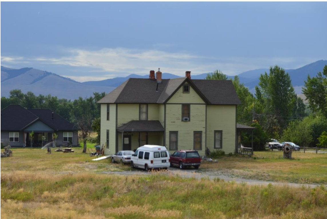
24MO0519, the Maclay House, west elevation, view to the east.
