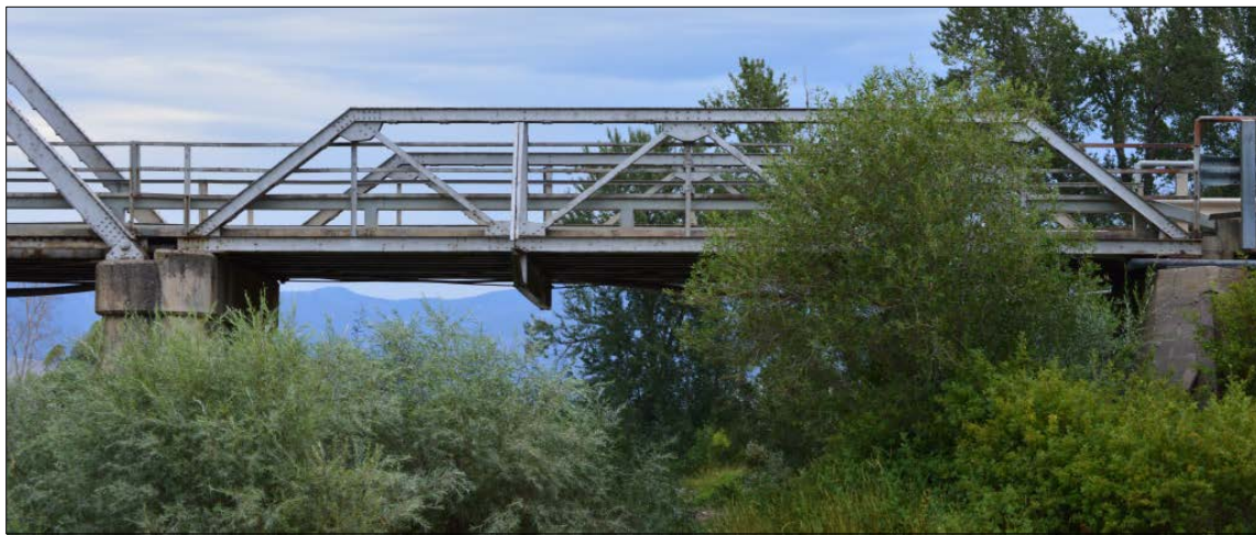
Figure 5-7. Warren truss section of the Maclay Bridge.
