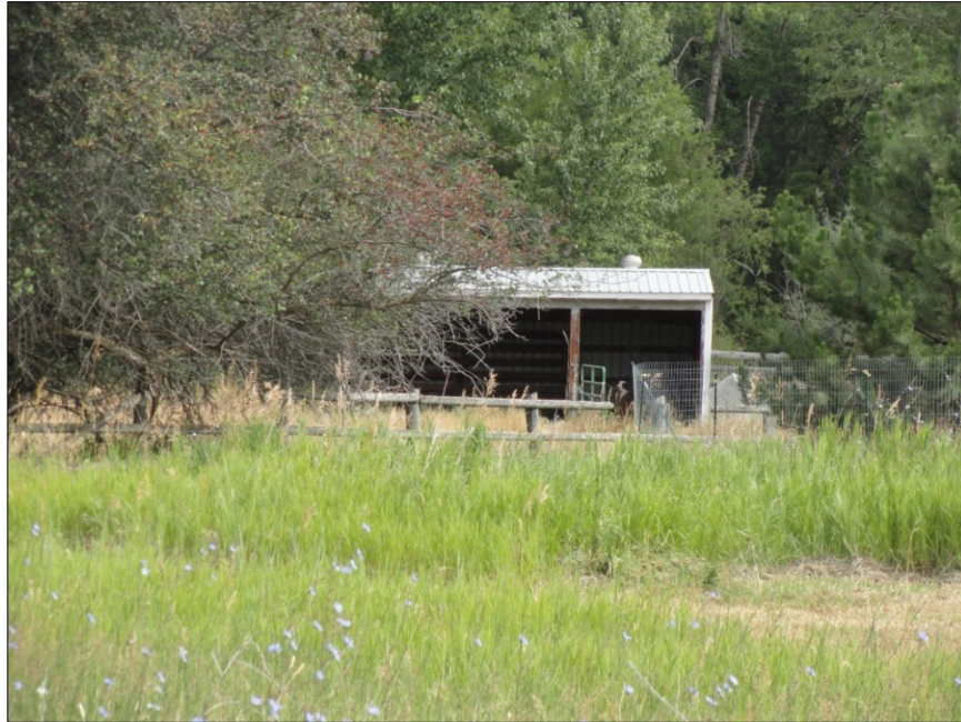
Figure 4-5. Overview of barn or storage shed #1, south elevation, view to the north.
