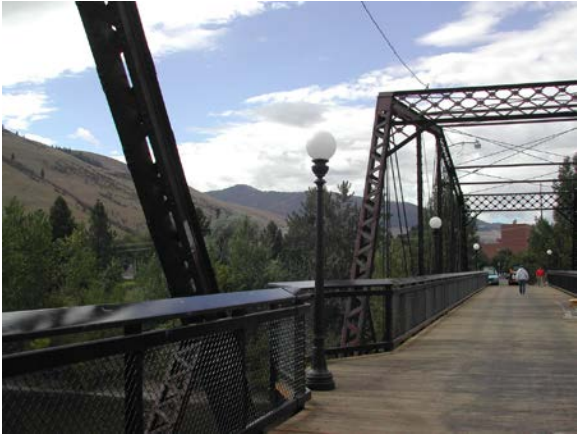
(Note: the above photos of the Pablo Pedestrian Bridge demonstrate examples of railings, not form liners – these abutments were faced in actual stone)
