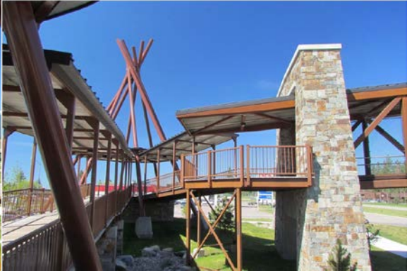
(Note: the above photos of the Pablo Pedestrian Bridge demonstrate examples of railings, not form liners – these abutments were faced in actual stone)
