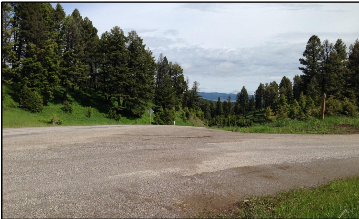
Photo 72. Looking at insufficient sight distance due to horizontal and vertical curves at the Battle Ridge campground access on MT 86. RP 20.5.
