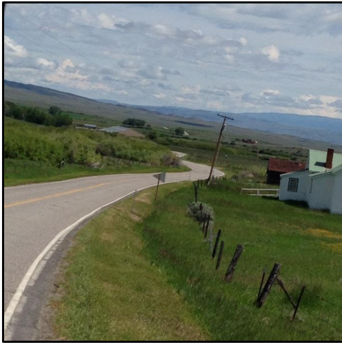
Photo 81. Looking at insufficient sight distance due to horizontal and vertical curves on MT 86. RP 26.8.
