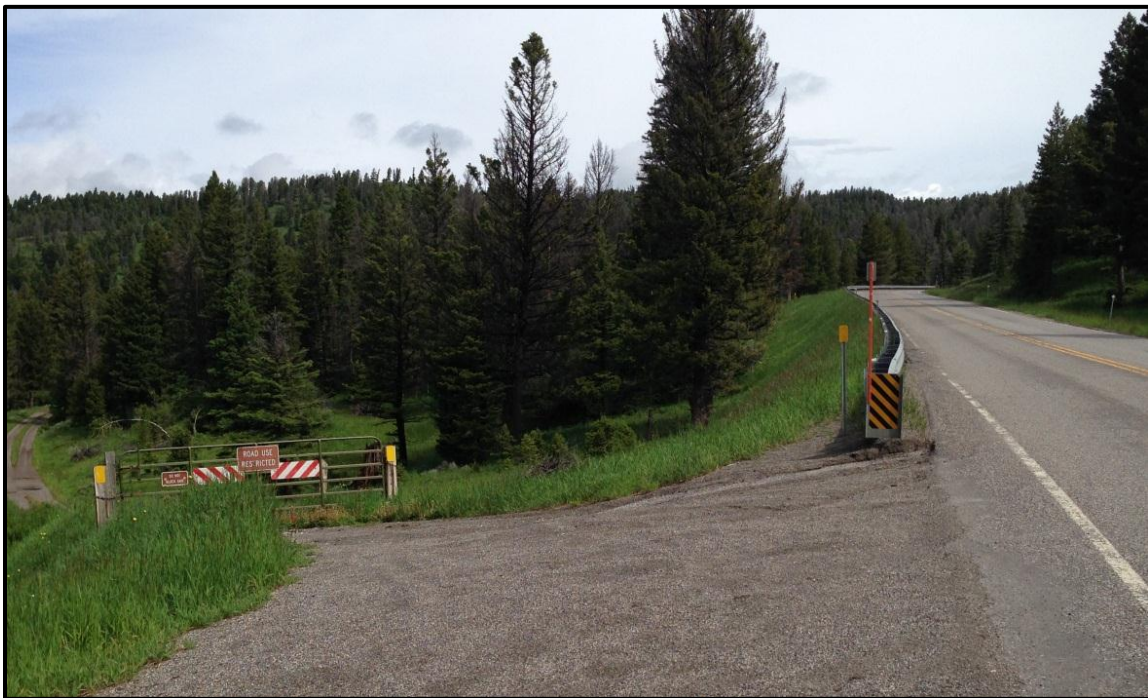
Photo 70. Looking at insufficient sight distance due to horizontal curves on MT 86. RP 19.5.
