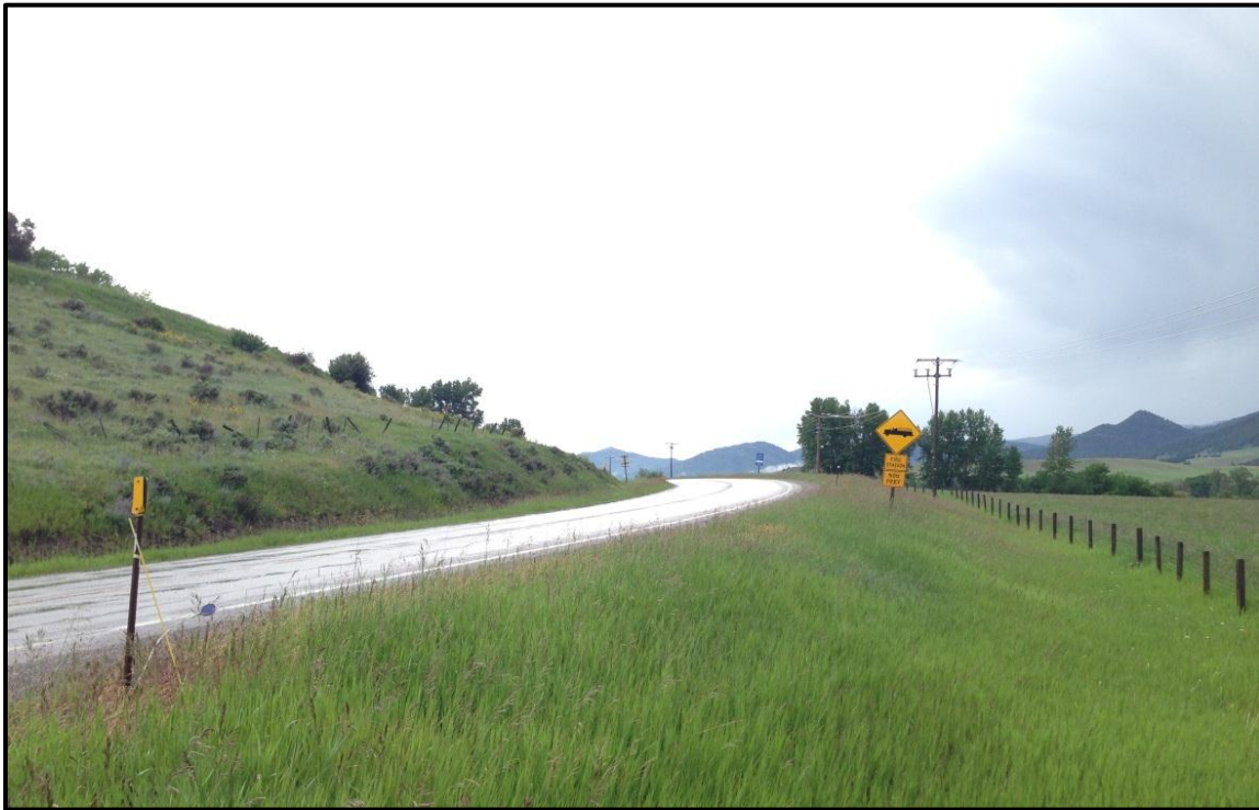
Photo 55. Looking at insufficient sight distance due to a horizontal curve on MT 86. RP 7.9.
