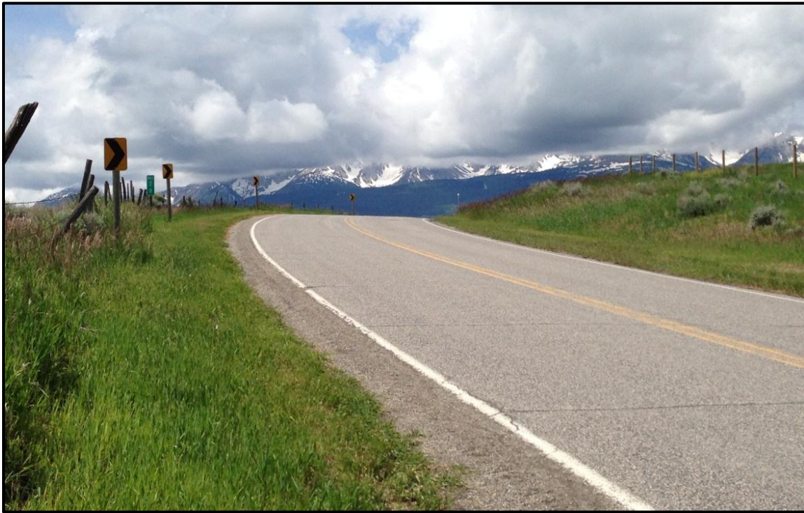
Photo 89. Looking south at insufficient sight distance due to horizontal and vertical curves on MT 86. RP 28.7.
