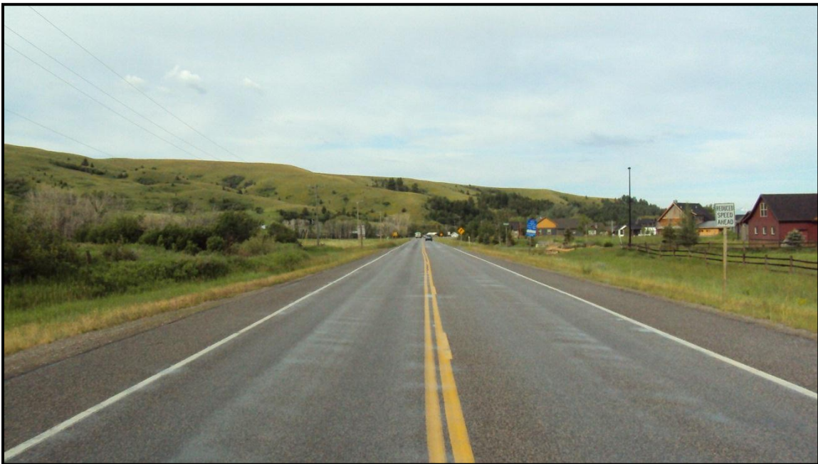
Photo 36. Looking south on MT 86 near the city limits of Bozeman. RP 3.0.
