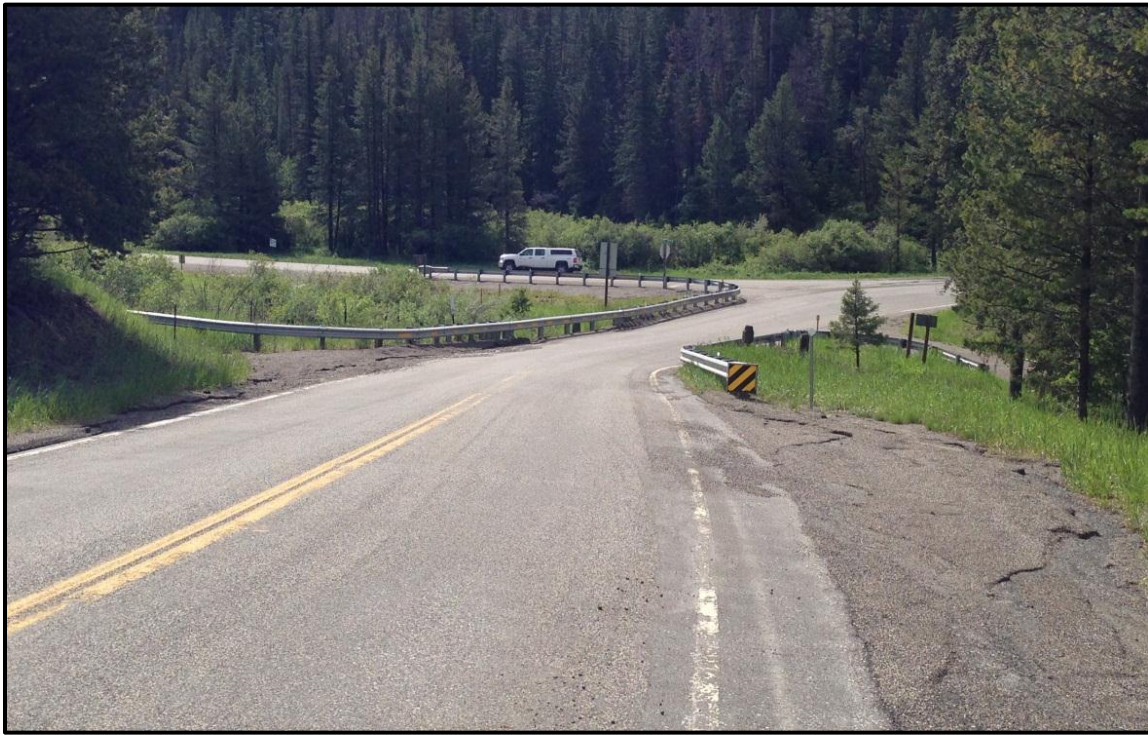
Photo 69. Looking at insufficient sight distance due to horizontal and vertical curves on MT 86 near Brackett Creek. RP 18.8.
