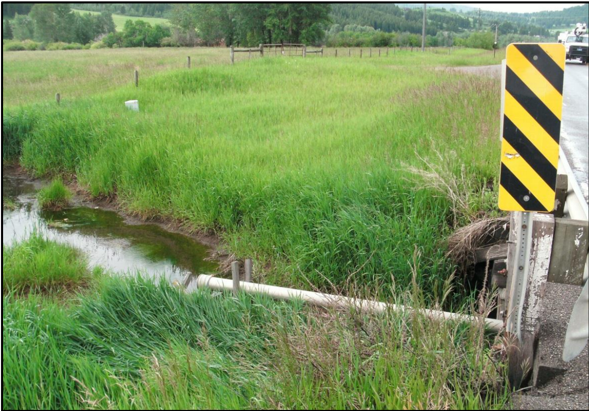
Photo 11. Looking downstream (south) at an unnamed tributary to Bridger Creek. RP 8.1.
