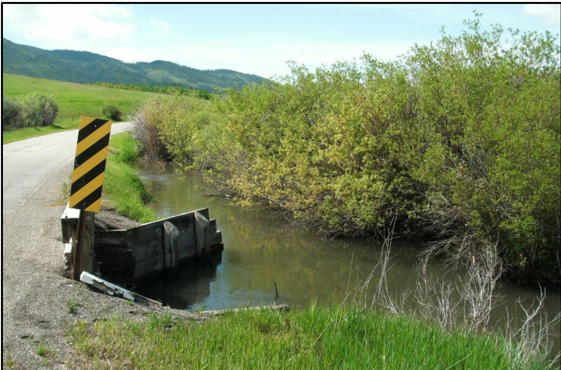
Photo 28. Looking upstream (southwest) on the MT 86 crossing of Cache Creek. RP 24.5.
