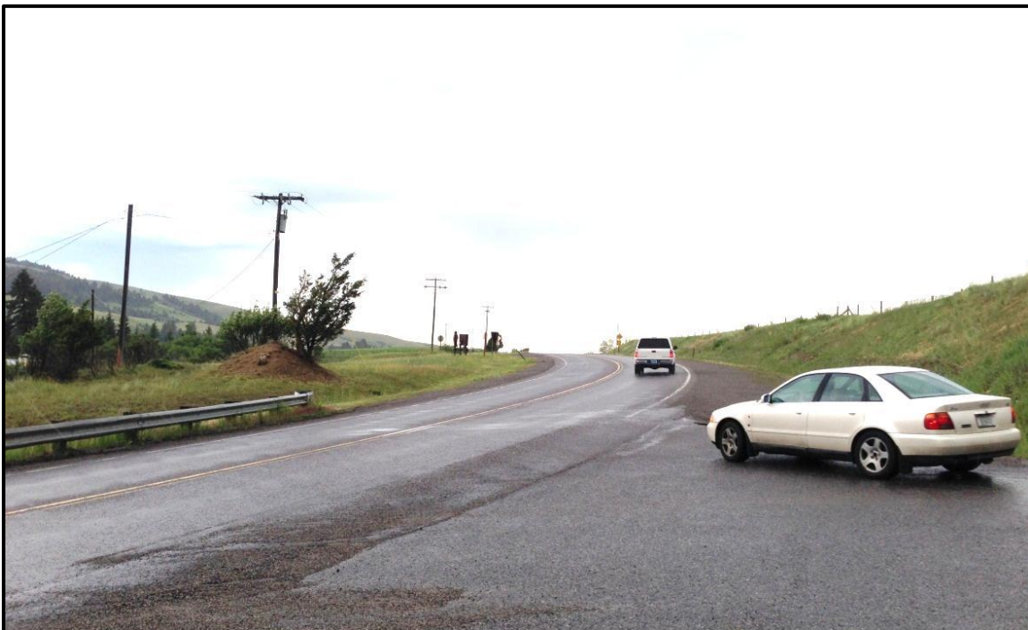
Photo 42. Looking north at insufficient sight distance due to vertical and horizontal curves on MT 86 at the access to "M" trail parking lot. RP 4.2.
