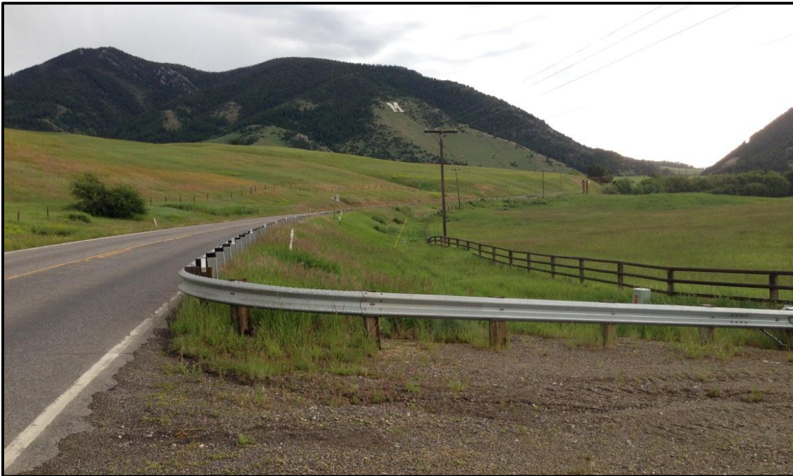
Photo 39. Looking at insufficient shoulder width along MT 86. RP 3.2.
