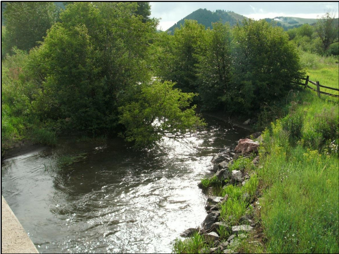
Photo 3. Looking upstream (south) on the MT 86 crossing of Bridger Creek. RP 3.1.
