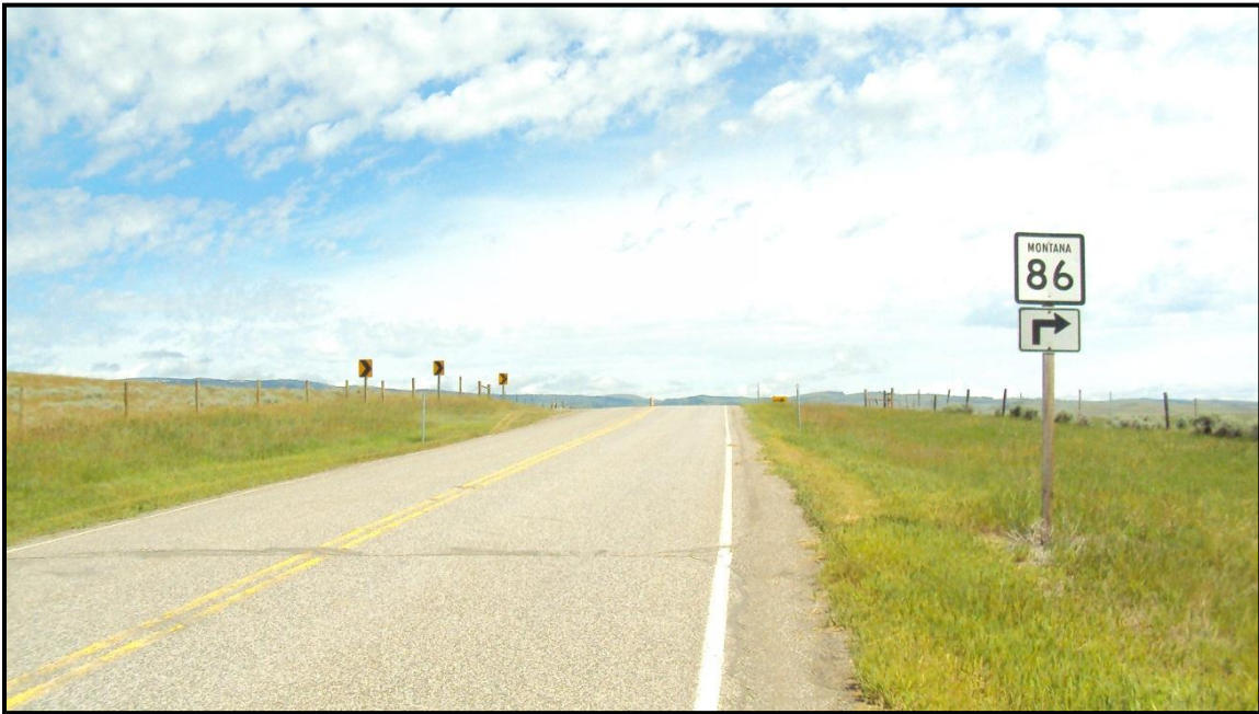
Photo 93. Looking north on MT 86, signage advises roadway users of a 90-degree turn. RP 28.8.
