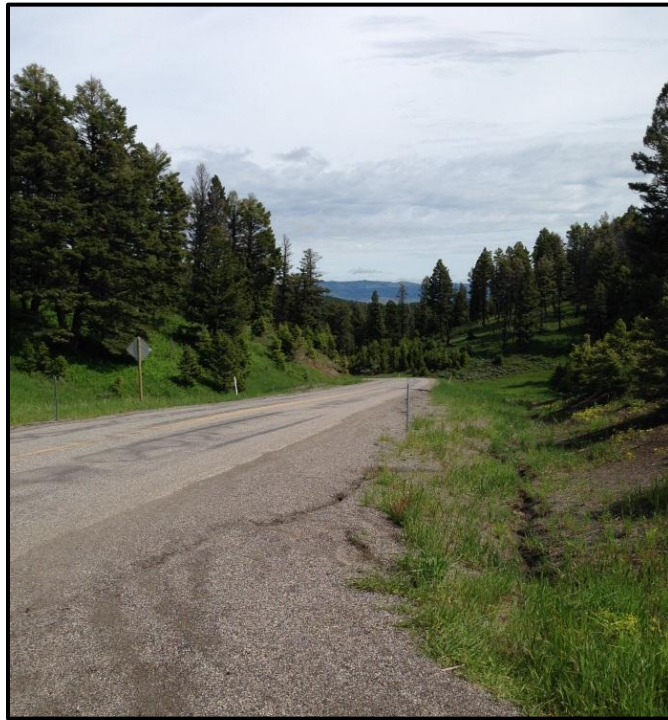
Photo 71. Looking at insufficient sight distance due to horizontal and vertical curves and steep grades on MT 86. RP 20.5.
