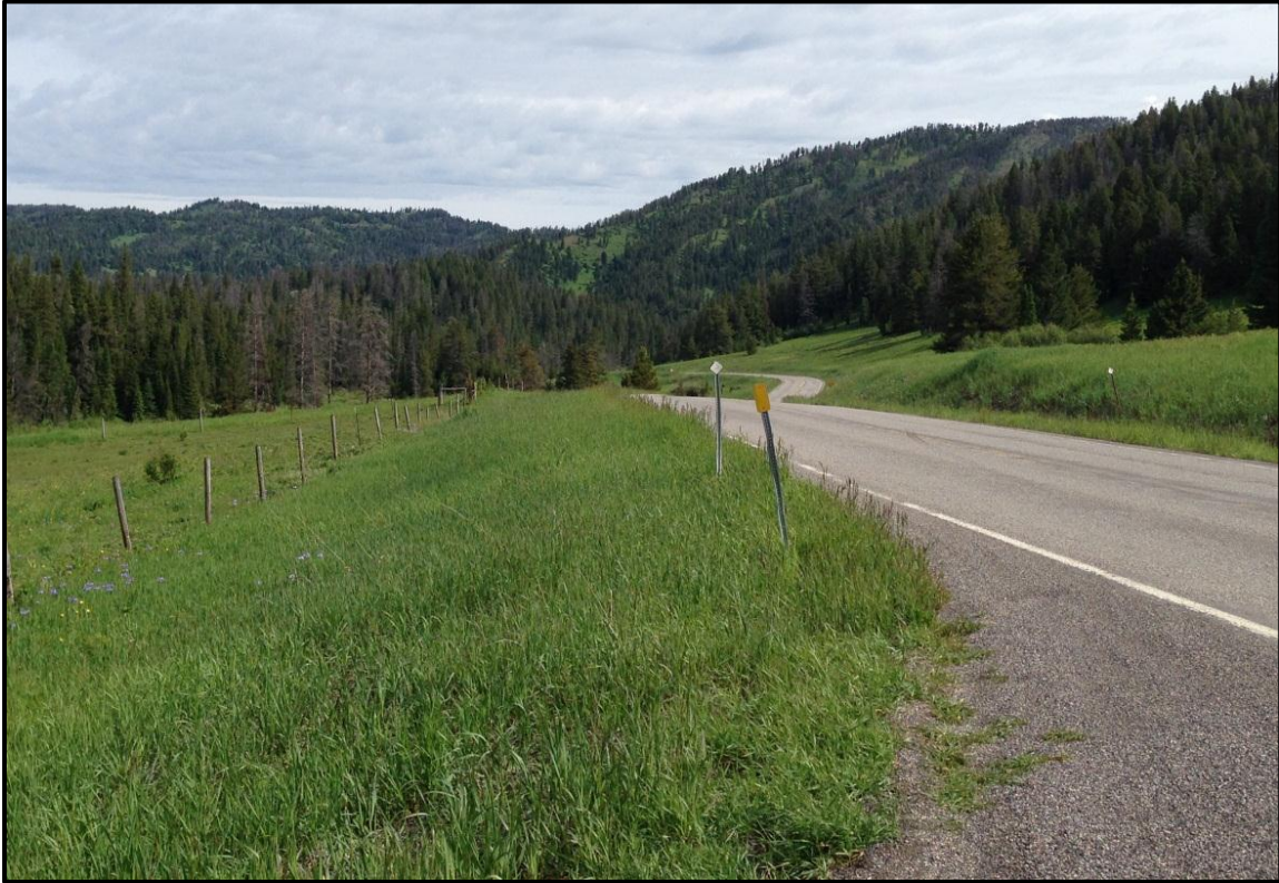
Photo 65. Looking at sight distance issues due to horizontal and vertical curves on MT 86. RP 17.9.
