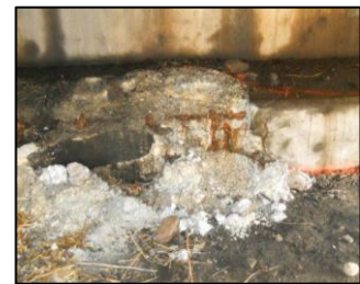
Concrete spalling is a form of surface failure resulting in splintered concrete chips and fragments.
