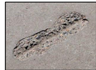
Concrete delamination is a form of surface failure resulting in separation of the surface layer.
