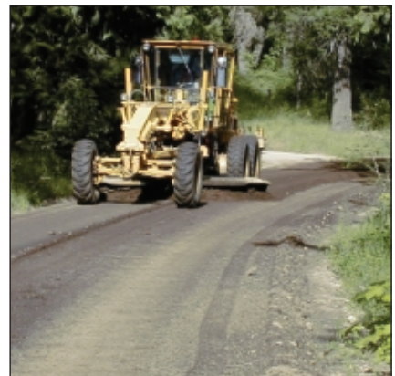
Figure 4. Grading after in-place processing
