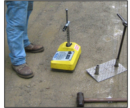
Figure 4: A Nuclear Density Meter calculates density and moisture.
