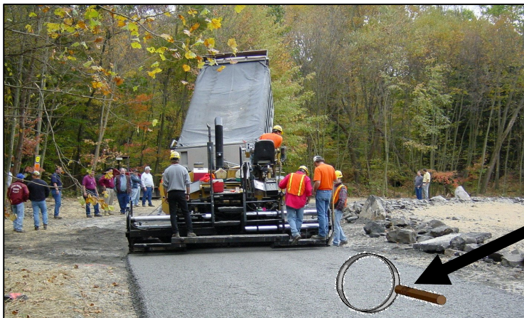
Figure 1: Placement of DSA through a paver.
