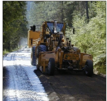
Figure 2. Blending with the in-place processor
