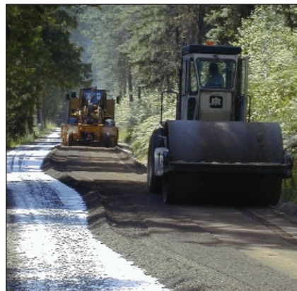
Figure 3. Compacting after in-place processing
