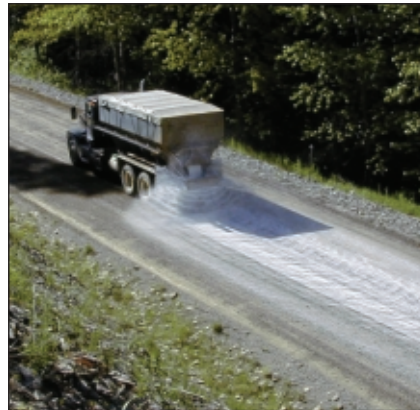
Figure 1. Spreading flake calcium chloride in one of the test sections.
