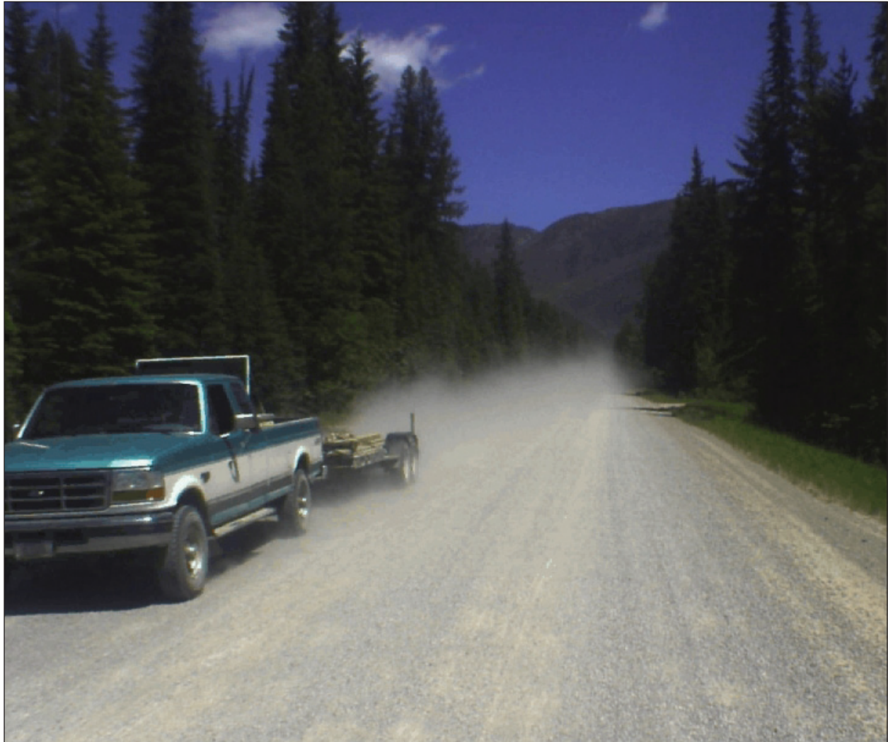
Figure 2.2 - Dust Rising Behind a Traveling Vehicle on the North Fork Flathead Road
