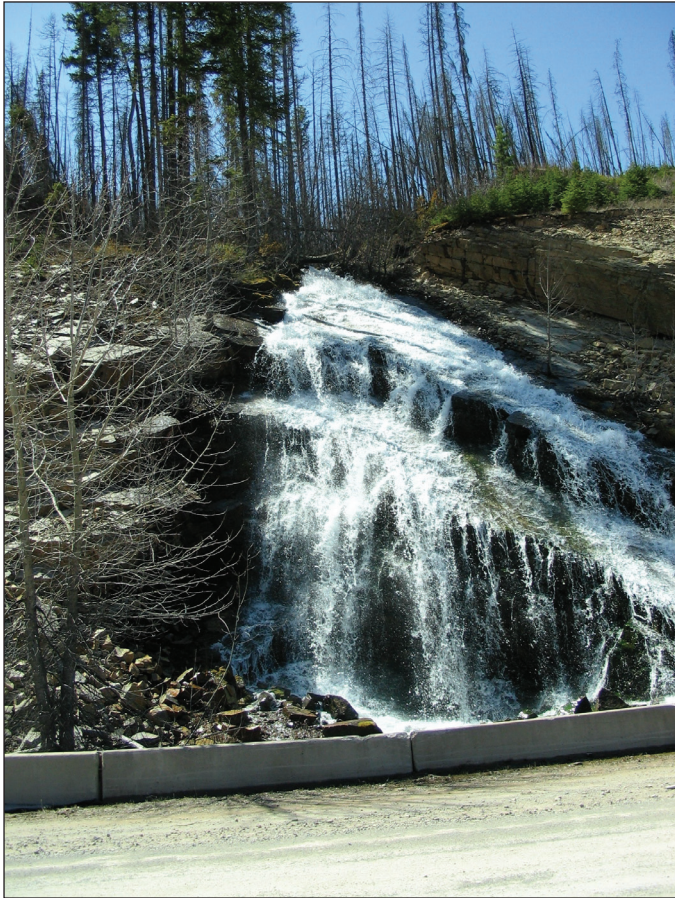
Figure 2.1 - Rock Face, Two Views on West Side of Highway 486
