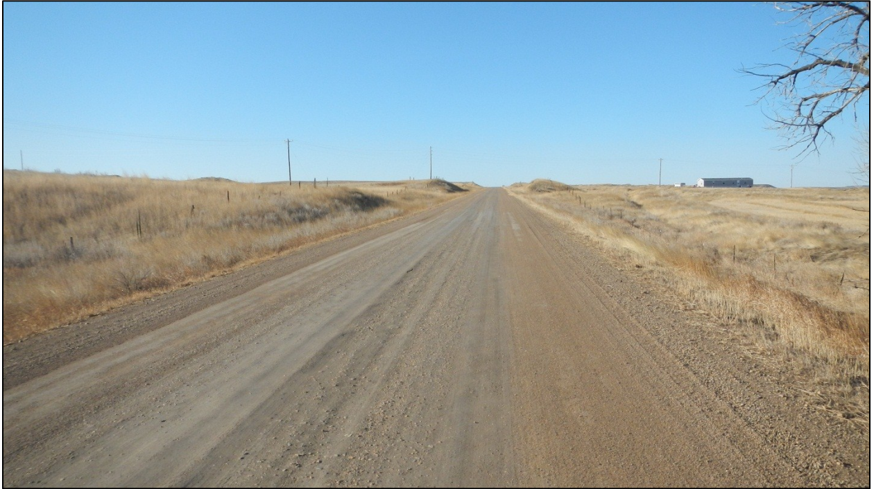
PHOTO 29: RP 21.0 LOOKING SOUTH
