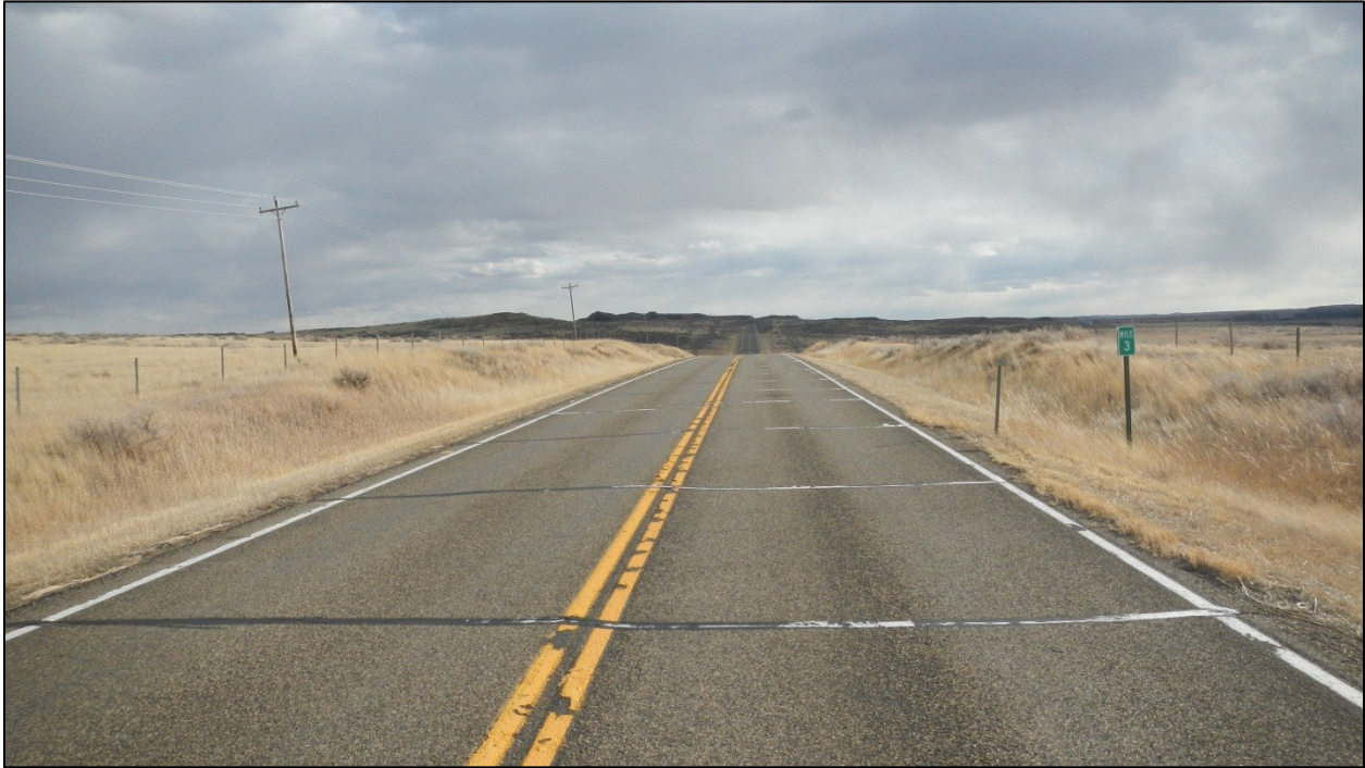
PHOTO 5: RP 3.0 LOOKING SOUTH
