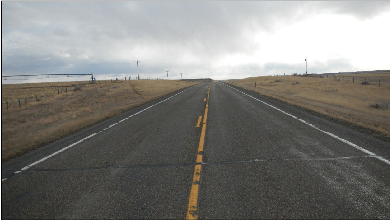
PHOTO 12: RP 6.0 LOOKING SOUTH
