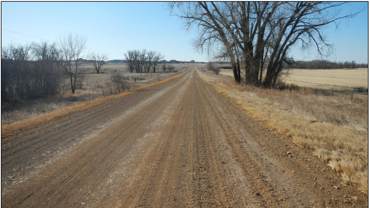
PHOTO 46: RP 35.0 LOOKING SOUTH
