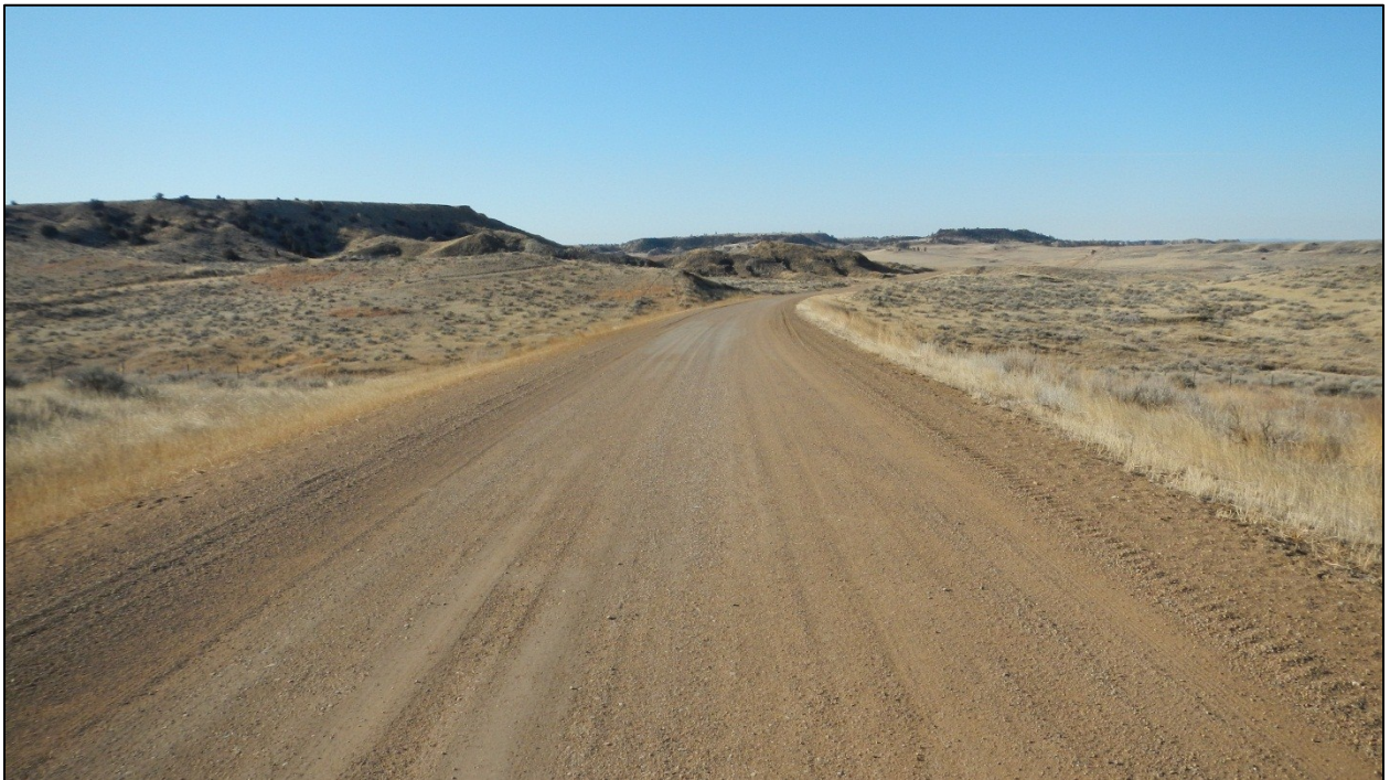
PHOTO 32: RP 24.0 LOOKING SOUTH
