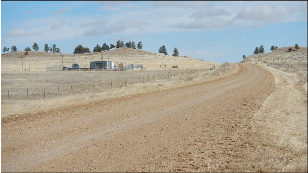
PHOTO 43: RP 32.5 LOOKING NORTH – PIPELINE TRANSMISSION BUILDING
