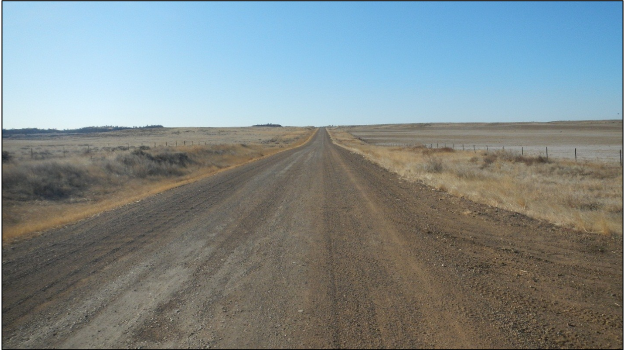
PHOTO 31: RP 23.0 LOOKING SOUTH
