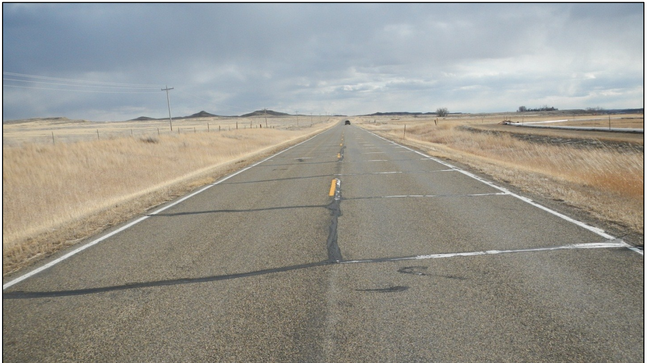
PHOTO 4: RP 2.0 LOOKING SOUTH
