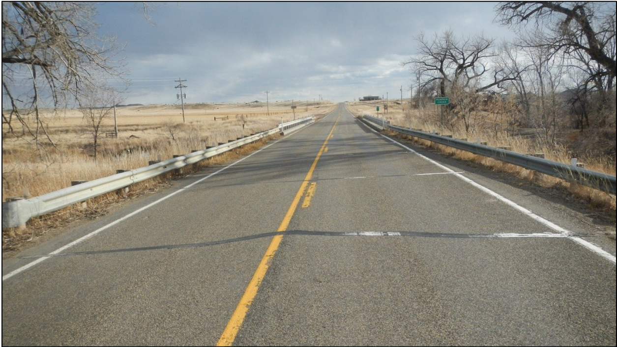
PHOTO 2: RP 1.0 LOOKING SOUTH – PUMPKIN CREEK BRIDGE
