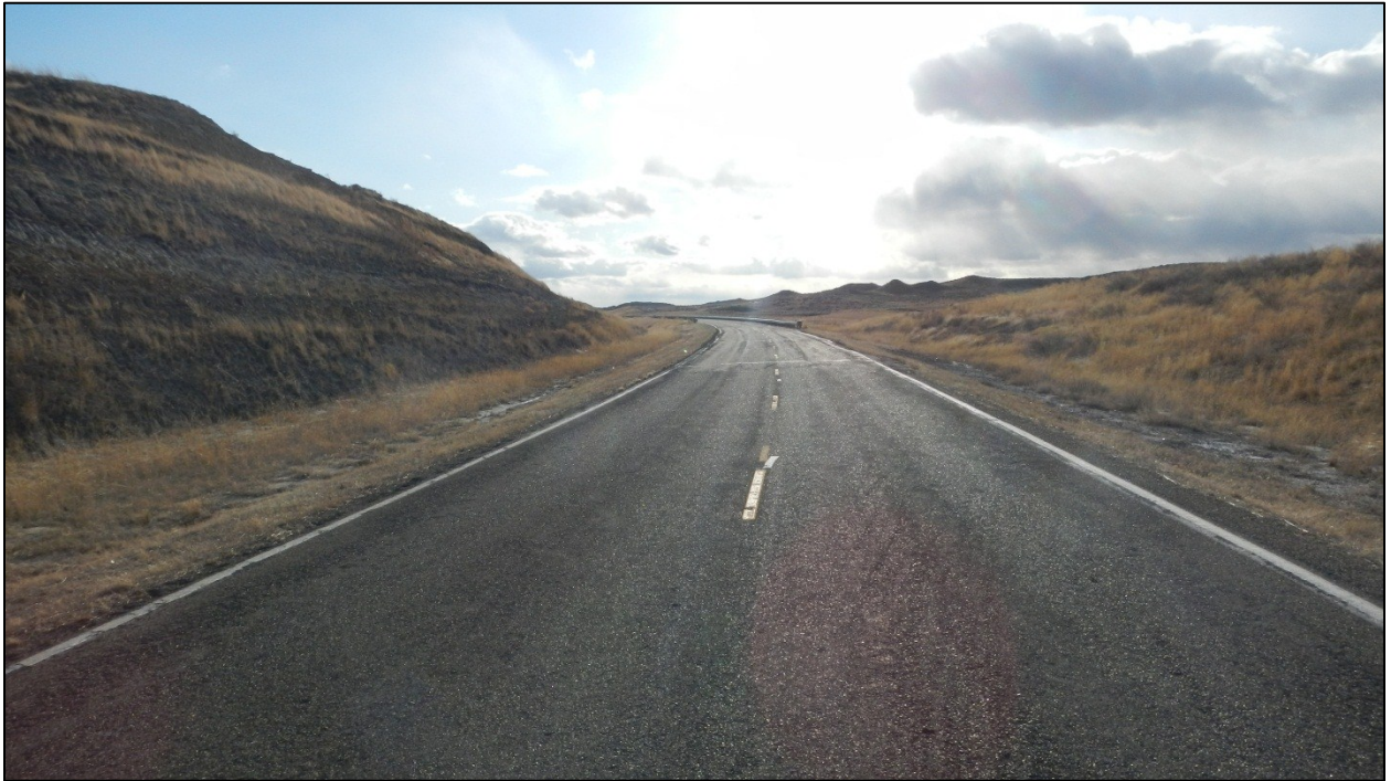
PHOTO 20: RP 14.0 LOOKING SOUTH
