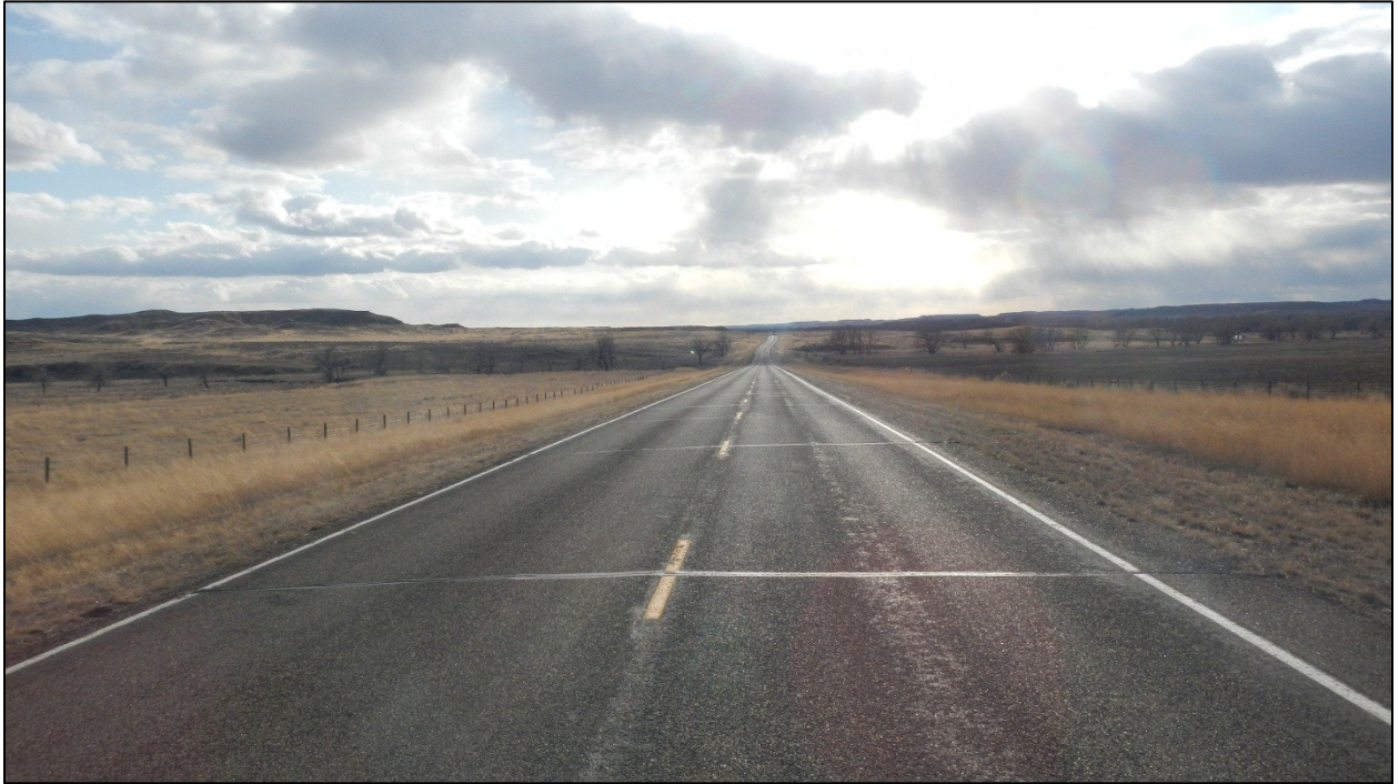
PHOTO 23: RP 17.0 LOOKING SOUTH
