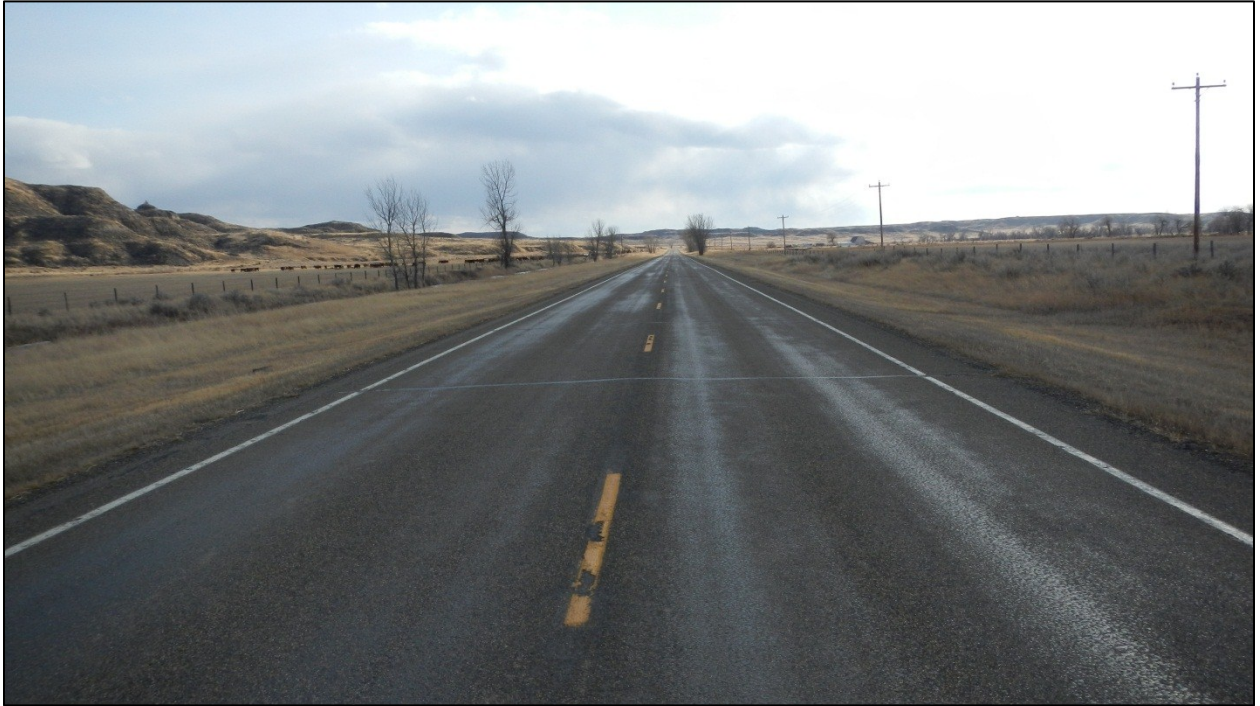
PHOTO 17: RP 11.0 LOOKING SOUTH
