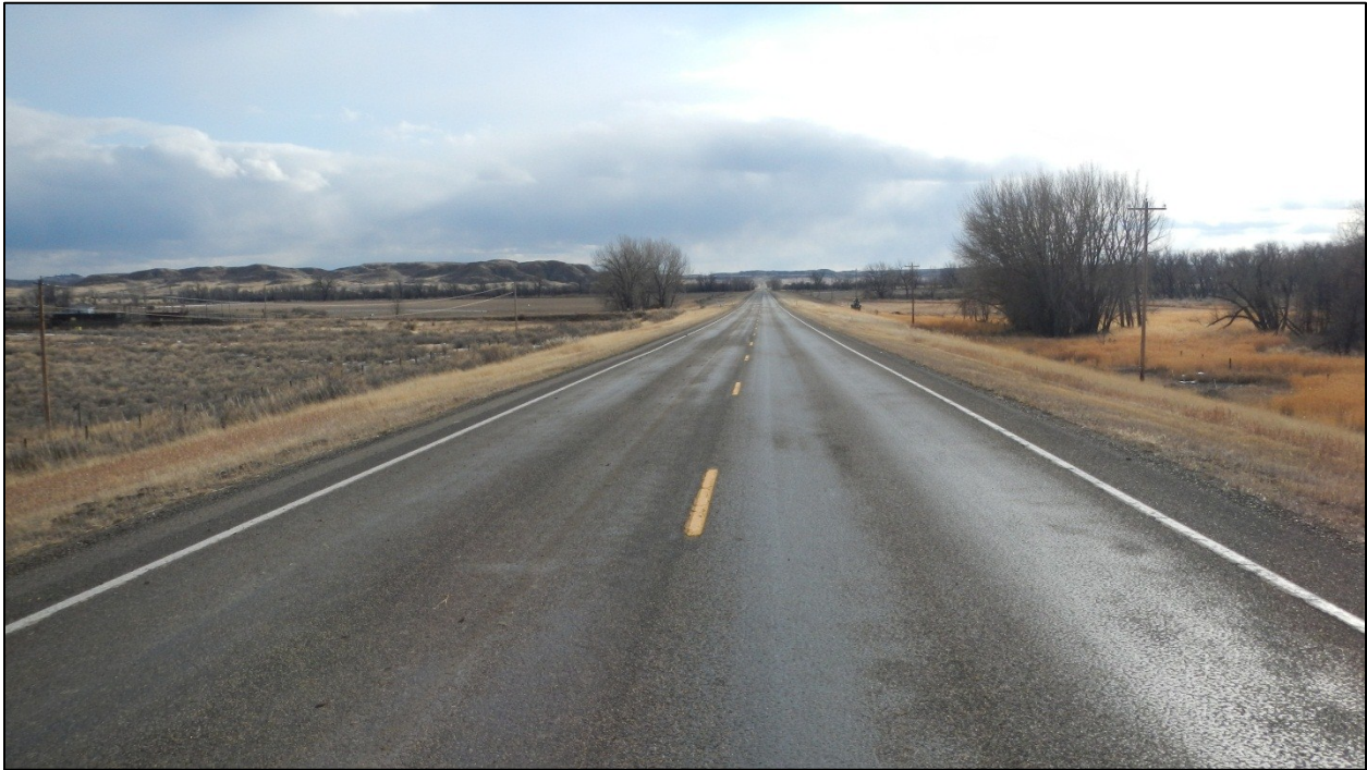
PHOTO 16: RP 10.0 LOOKING SOUTH
