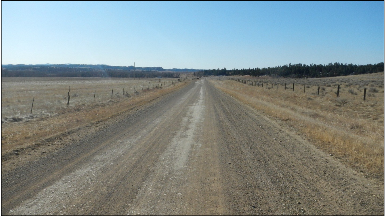
PHOTO 55: RP 42.0 LOOKING SOUTH
