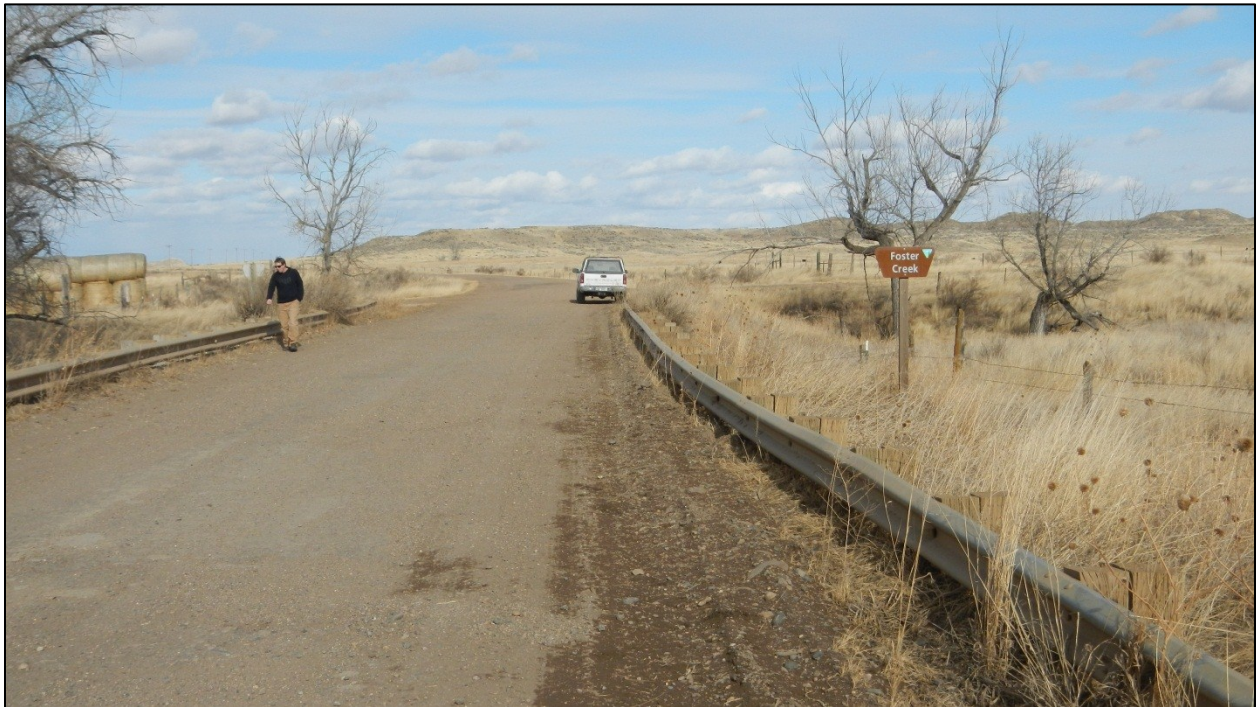
PHOTO 27: RP 19.9 LOOKING NORTH - FOSTER CREEK BRIDGE
