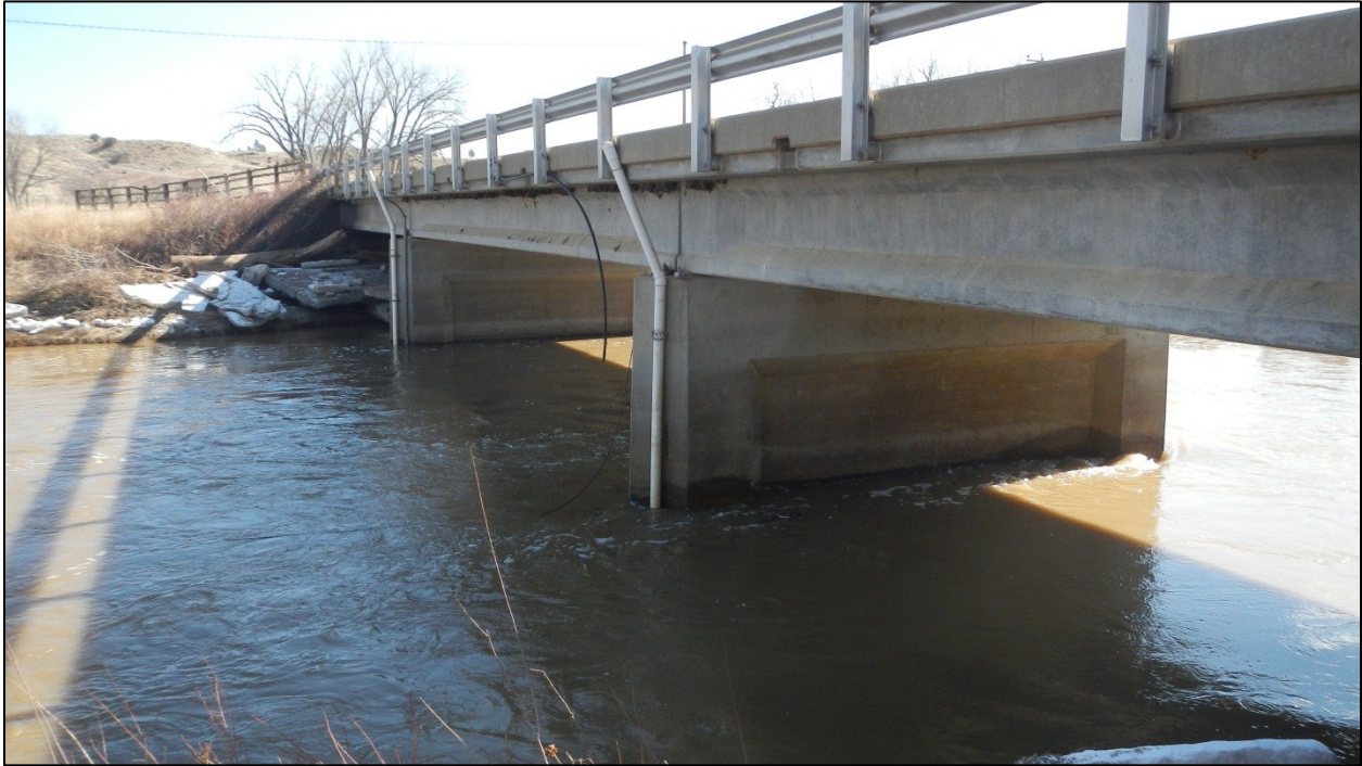
PHOTO 51: RP 39.6 LOOKING EAST - TONGUE RIVER BRIDGE
