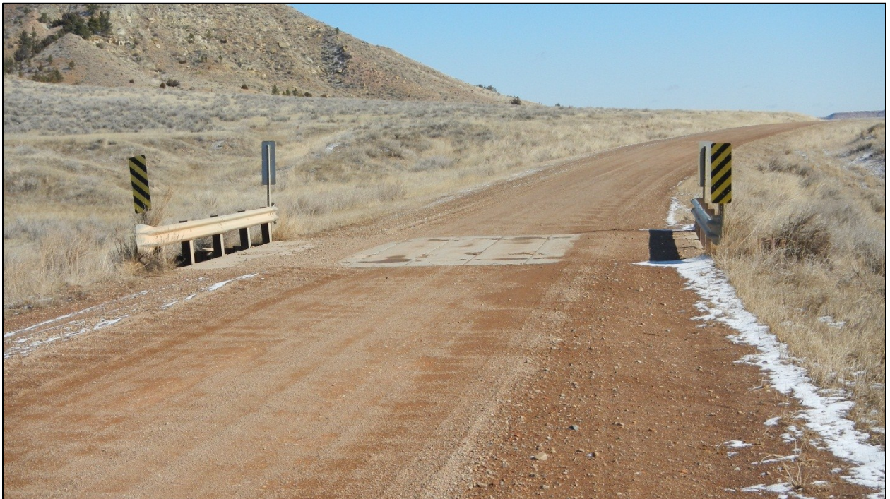
PHOTO 62: RP 47.8 LOOKING NORTHEAST - UNNAMED DRAINAGE BRIDGE
