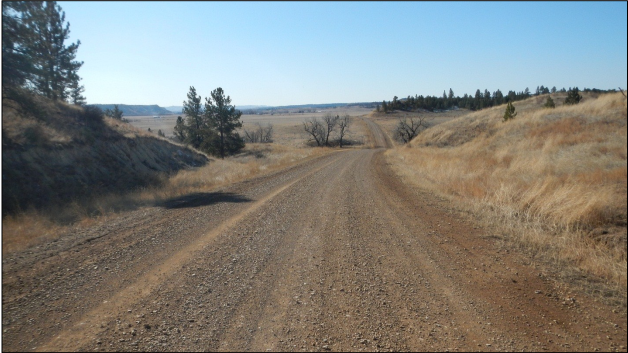
PHOTO 65: RP 50.0 LOOKING SOUTH
