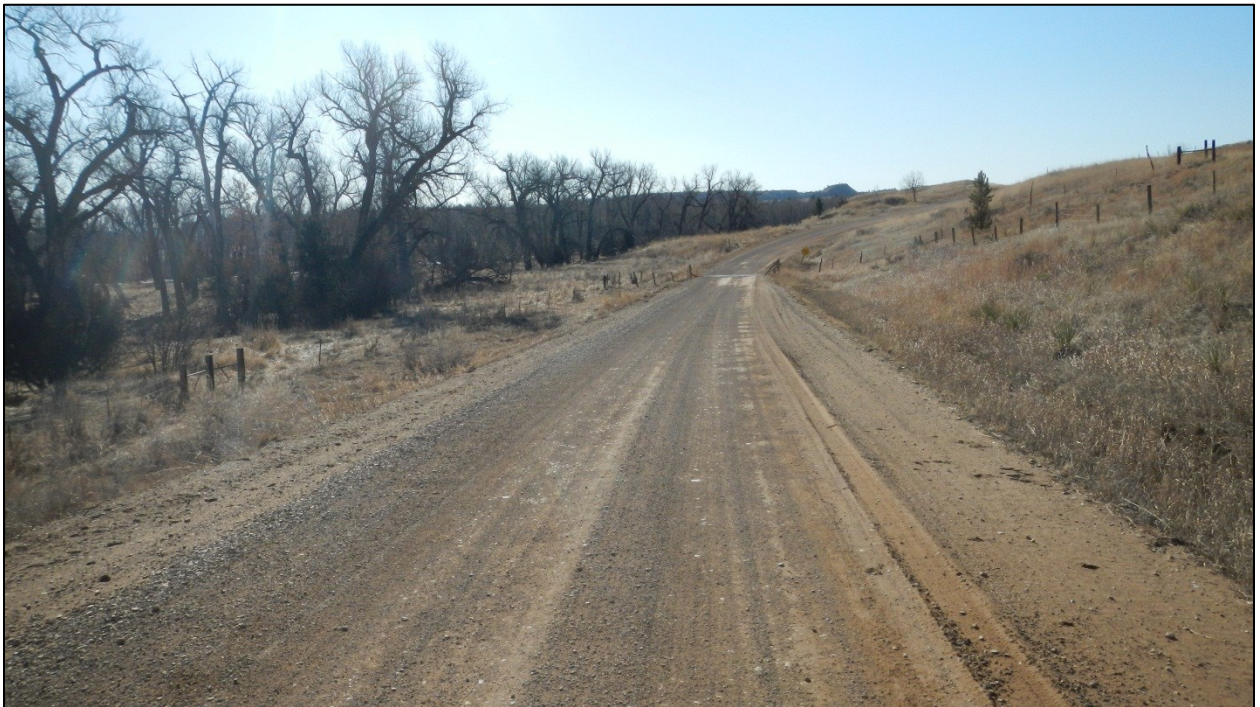
PHOTO 56: RP 43.0 LOOKING SOUTH
