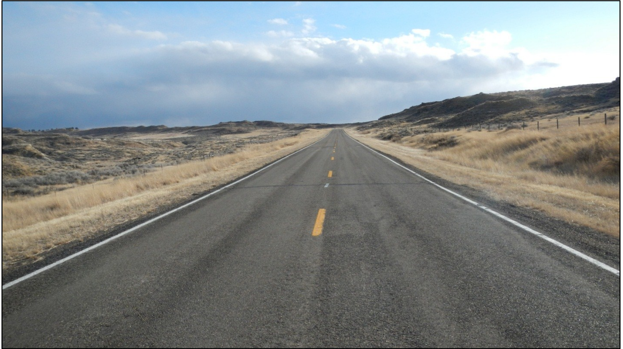
PHOTO 19: RP 13.0 LOOKING SOUTH
