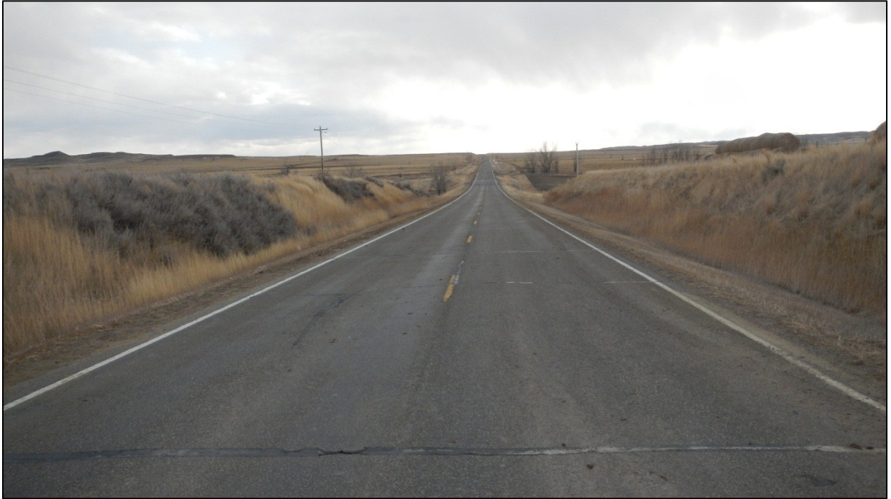
PHOTO 11: RP 5.0 LOOKING SOUTH
