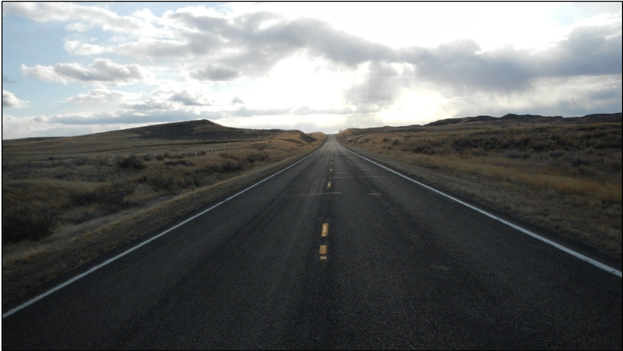
PHOTO 22: RP 16.0 LOOKING SOUTH
