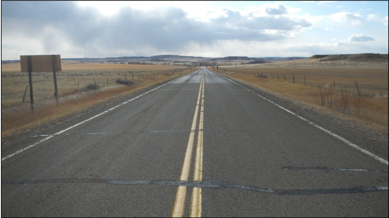
PHOTO 1: RP 0.0 LOOKING SOUTH
