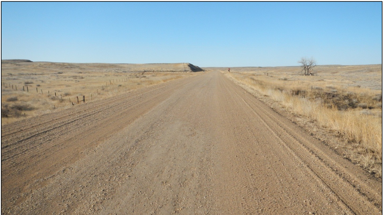
PHOTO 30: RP 22.0 LOOKING SOUTH
