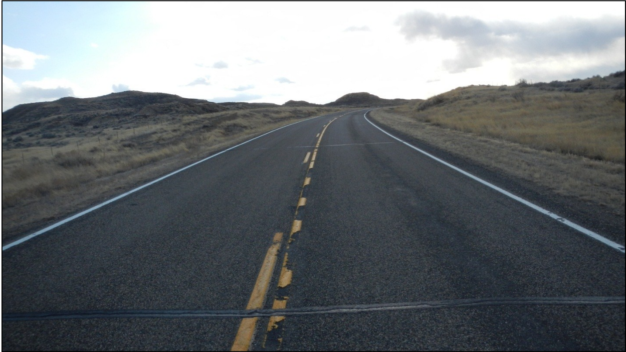
PHOTO 21: RP 15.0 LOOKING SOUTH
