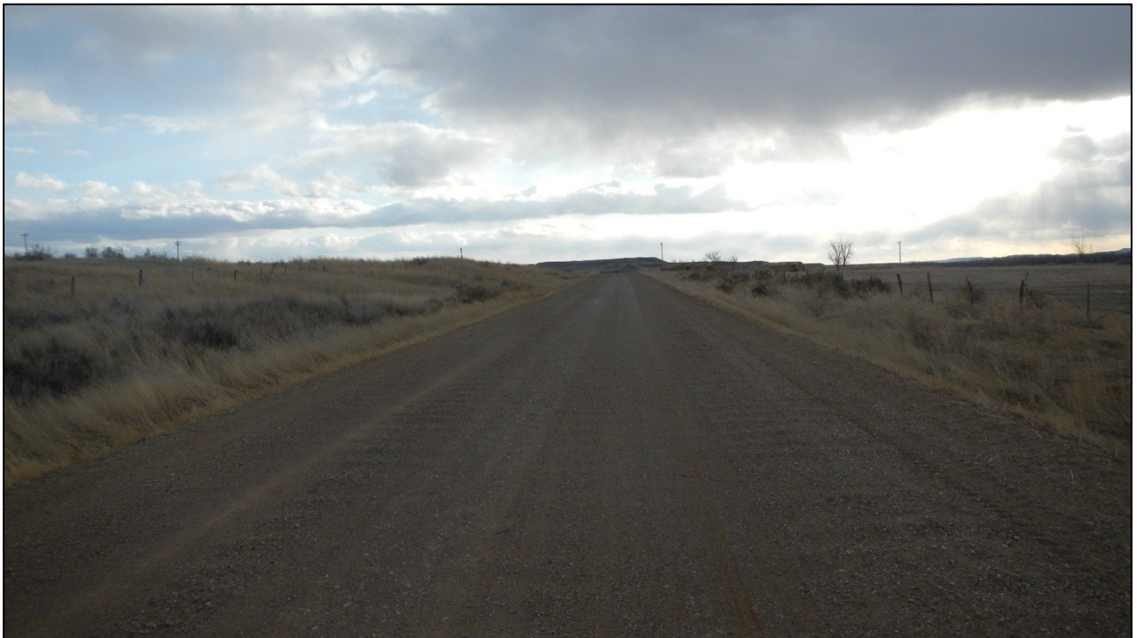
PHOTO 26: RP 19.0 LOOKING SOUTH
