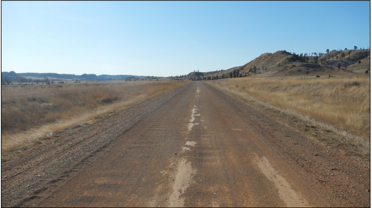
PHOTO 63: RP 48.0 LOOKING SOUTH
