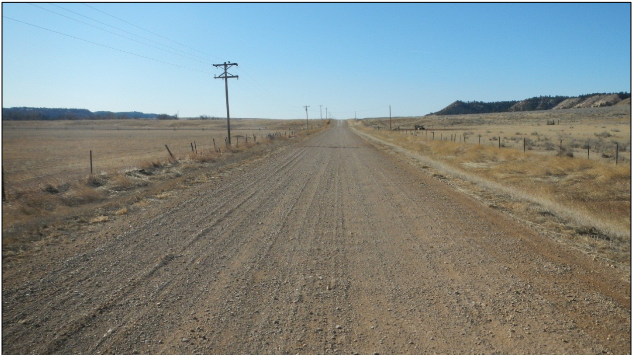
PHOTO 58: RP 45.0 LOOKING SOUTH
