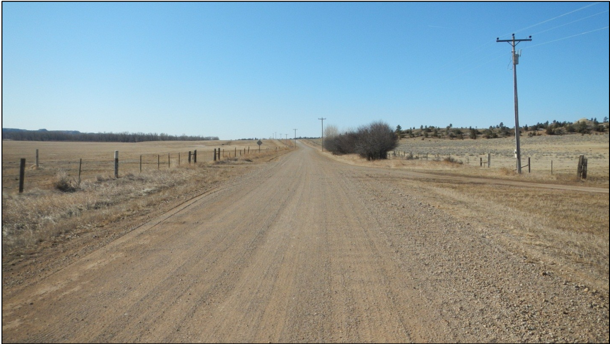
PHOTO 54: RP 41.0 LOOKING SOUTH
