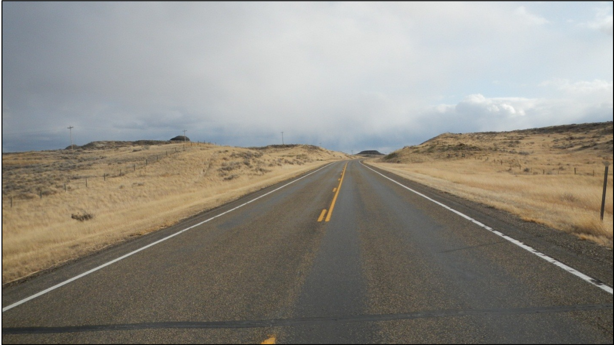
PHOTO 15: RP 9.0 LOOKING SOUTH
