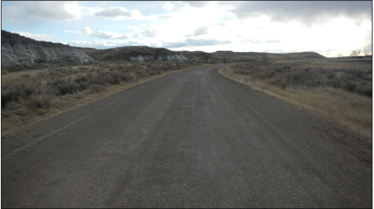
PHOTO 25: RP 18.0 LOOKING SOUTH
