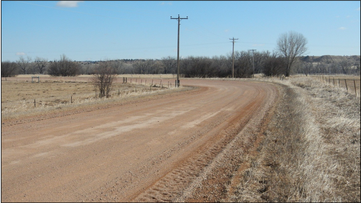
PHOTO 53: RP 40.7 LOOKING EAST - SUBSTANDARD HORIZONTAL CURVE
