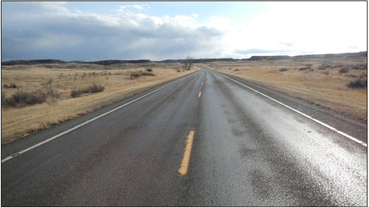
PHOTO 18: RP 12.0 LOOKING SOUTH
