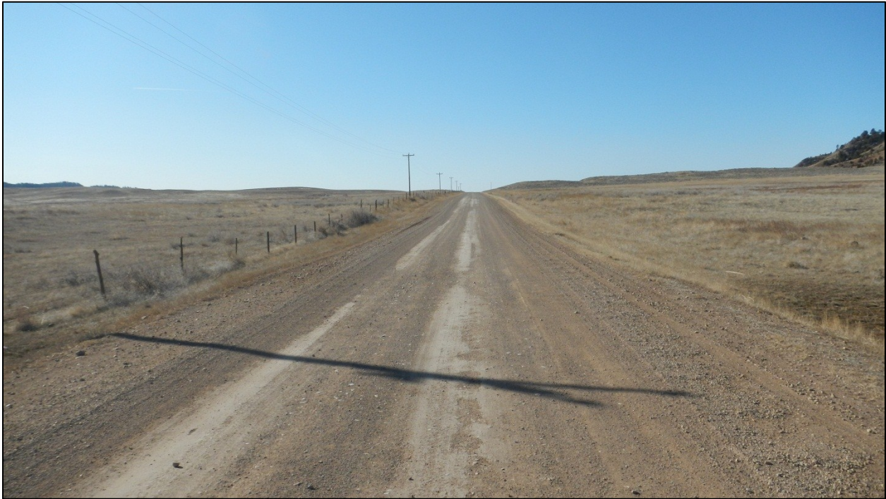
PHOTO 60: RP 46.0 LOOKING SOUTH
