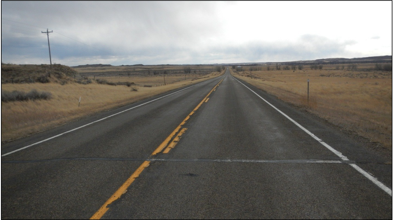
PHOTO 13: RP 7.0 LOOKING SOUTH
