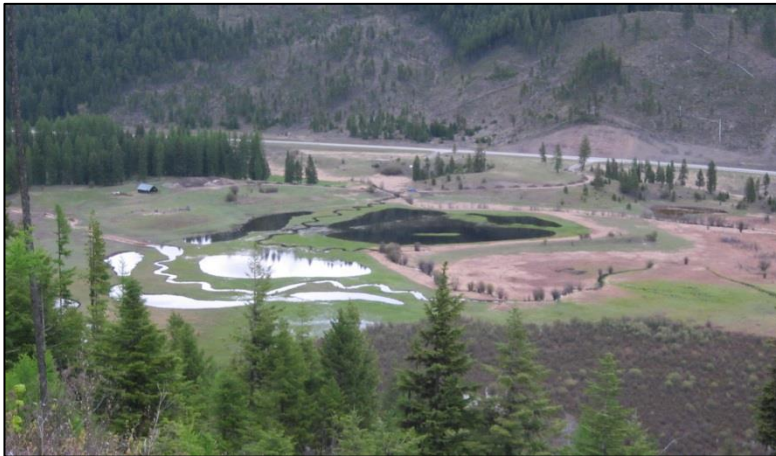
In 2014, MDT restored a large portion of the Schrieber Lake site, including segments of both Schrieber Creek and Coyote Creek
