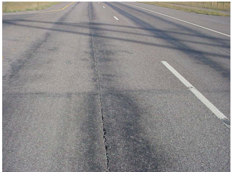
Figure 10: Longitudinal Crack
