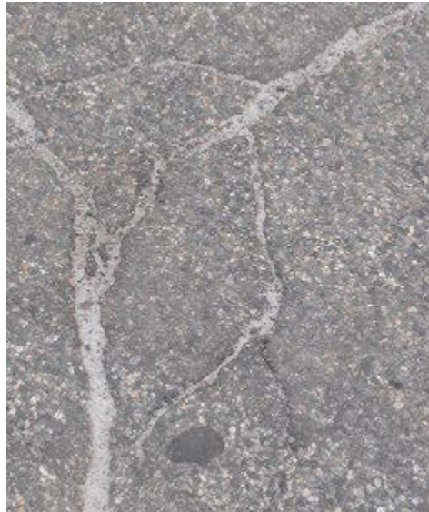
Figure 11: Secondary Crack
