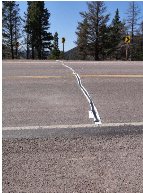
Figure 12: Transverse crack
