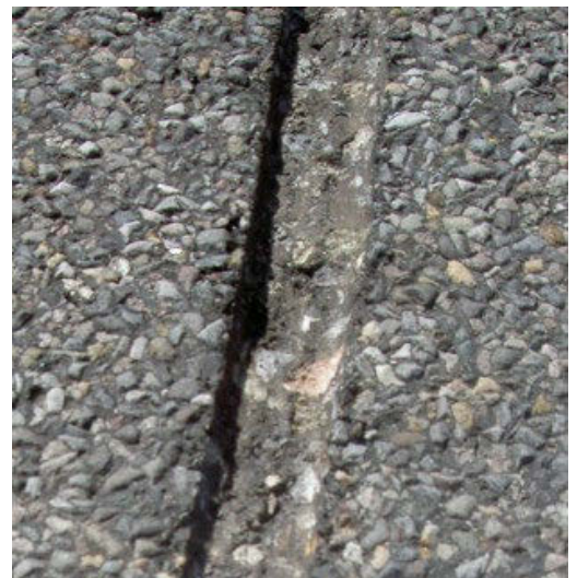
Figure 8: Routed crack
