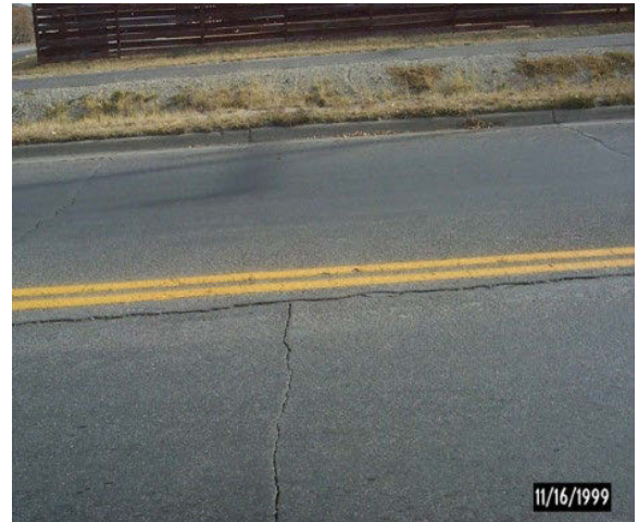
Figure 2 Transverse/Longitudinal cracking
