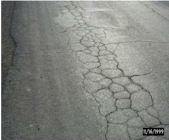
Figure 1 Alligator cracking
