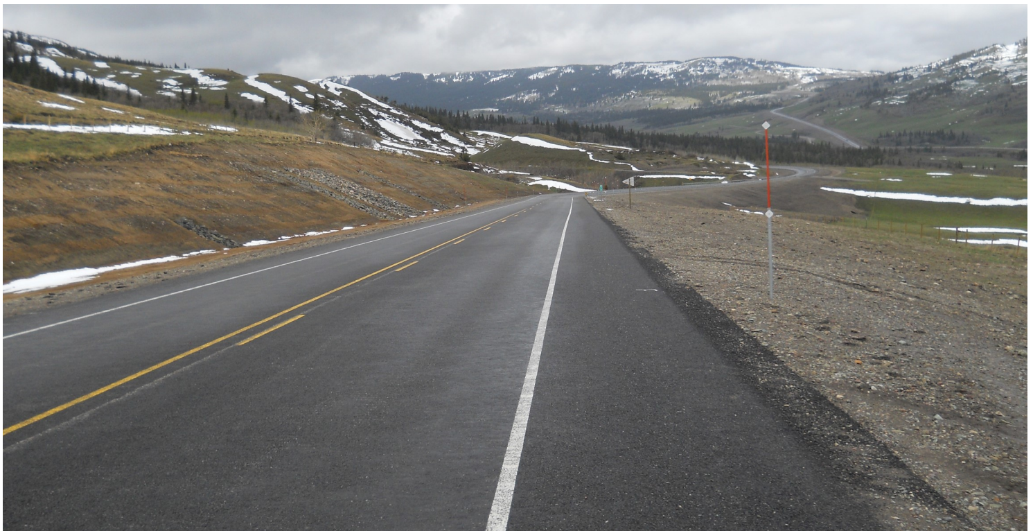
A picture taken of the completed North of Kiowa—North Project in 2020 on US Highway 87 between Browning and East Glacier Park.
