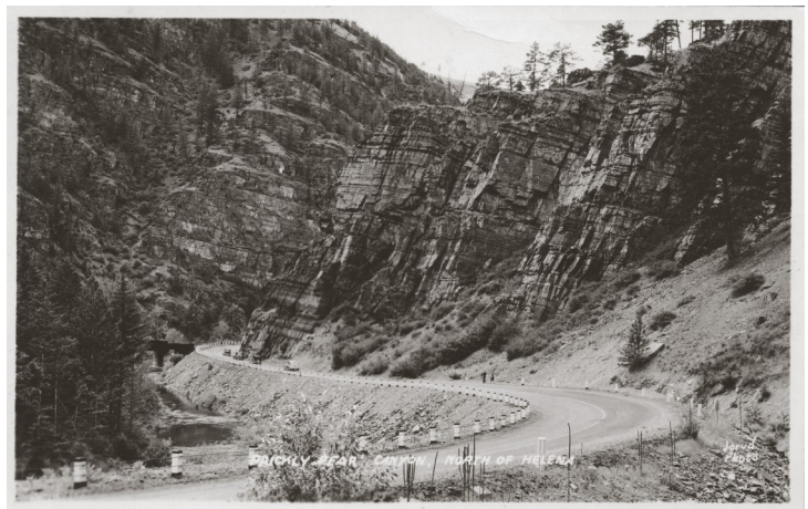
Construction progress along US-91 in Wolf Creek Canyon in the 1930's.
