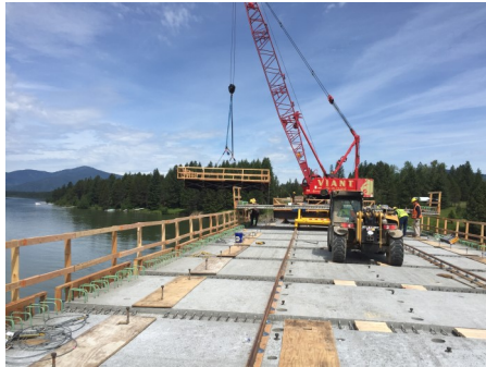
The Trout Creek bridge rehabilitation project (formally known as the Clark Fork River Bridge—1 Mile Northwest of Trout Creek and completed in late 2020) was the first in MDT history to use the CM/GC contracting method.
