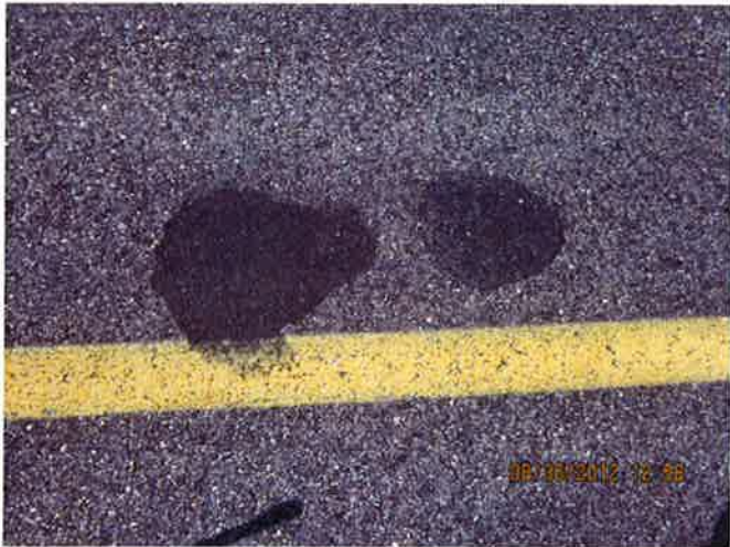
T-5, Surface detail with oil spillage
