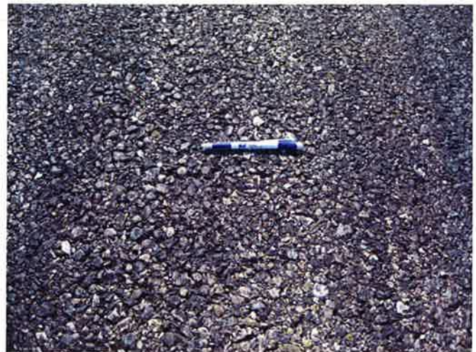
R-3, Surface detail with raveling
