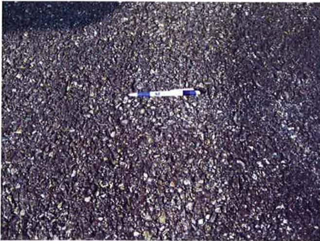
A-4, Surface detail with weathering
