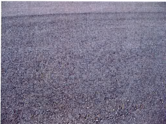
A-3, Surface detail with weathering
