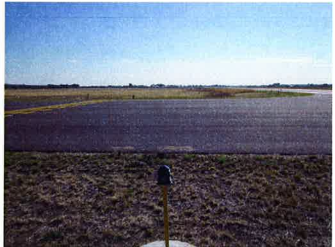
T-2, Turnaround overview
