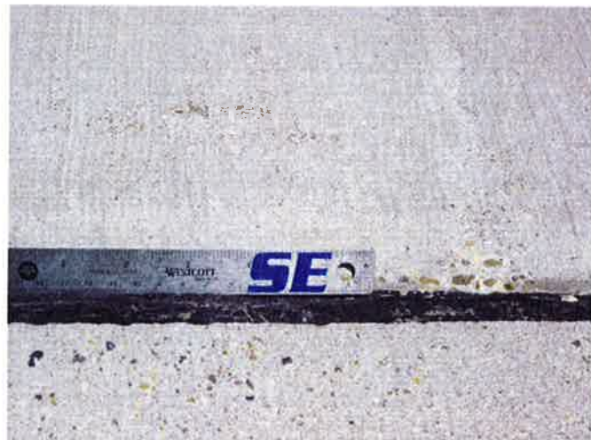
A-3, Surface detail of joint
