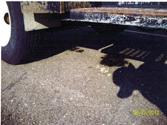
T-2, Oil spillage
