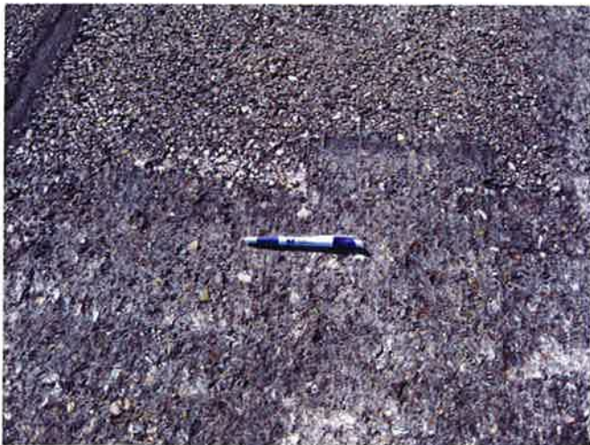
T-11, Surface detail with depression
