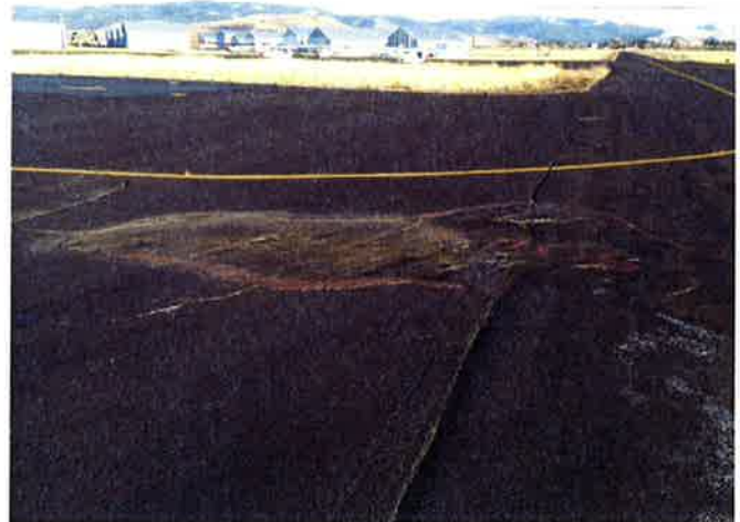
A-2 and T-3, Overview with depression
