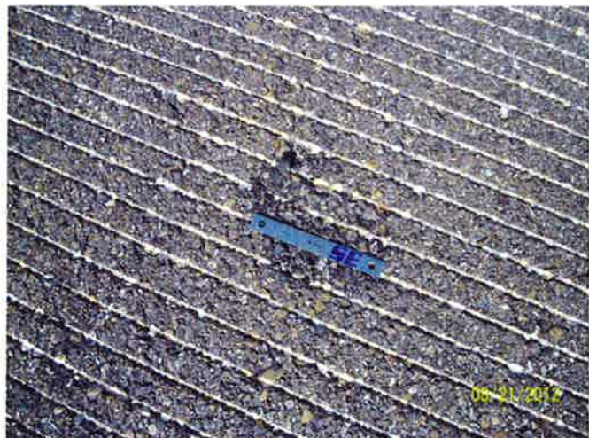
R-11, Surface detail raveling from lock wheel turn
