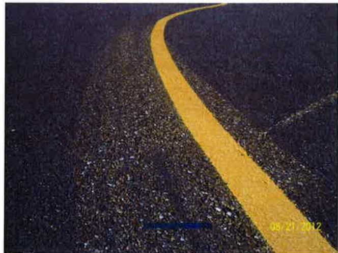
A-5, Surface detail raveling from paint obliteration
