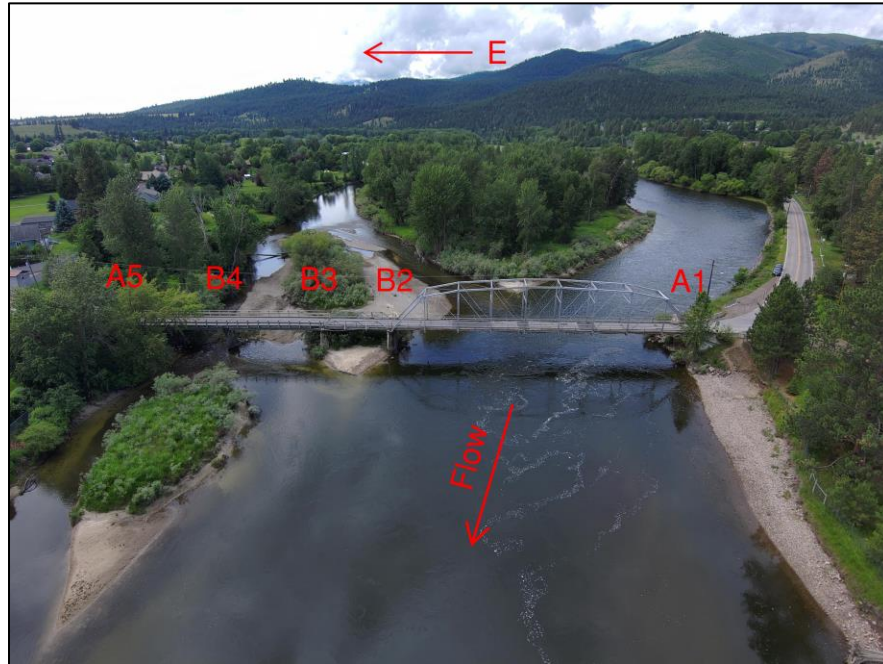
Photo 1: North Elevation looking south
