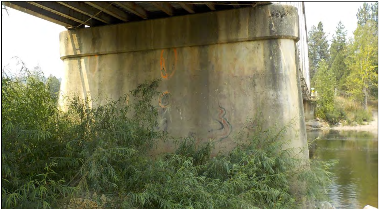
Photo 14: Bent 2 East Elevation looking west
