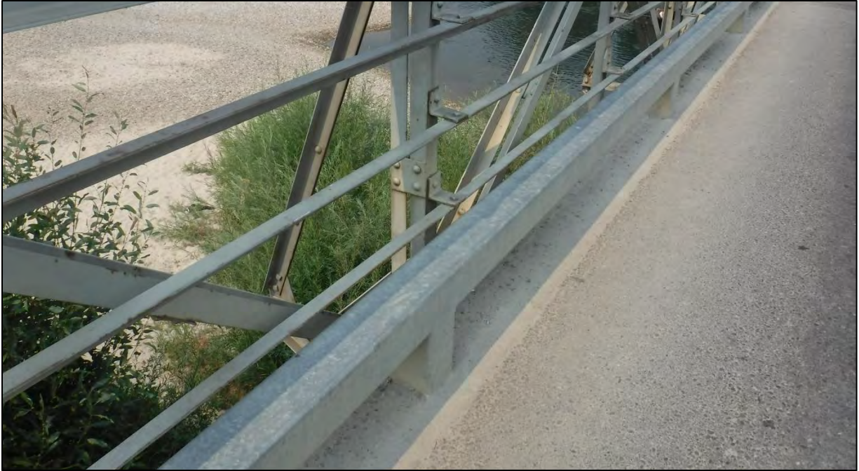
Photo 32: Bridge rail for Spans 1 and 2
