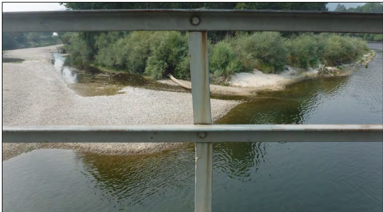
Photo 33: The vertical angle on the South Rail between Panel Point 4' and 3' was bent 1-1/2 in. over a 2 ft. length due to impact damage
