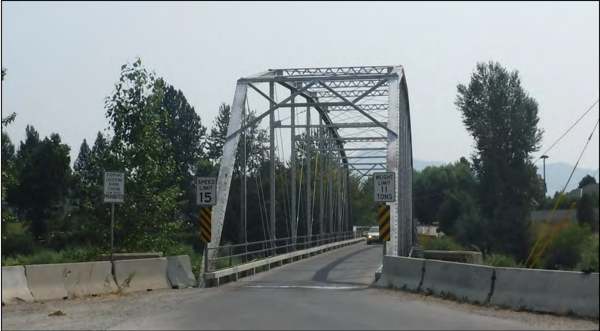
Photo 7: West Portal with Weight Limit Sign
