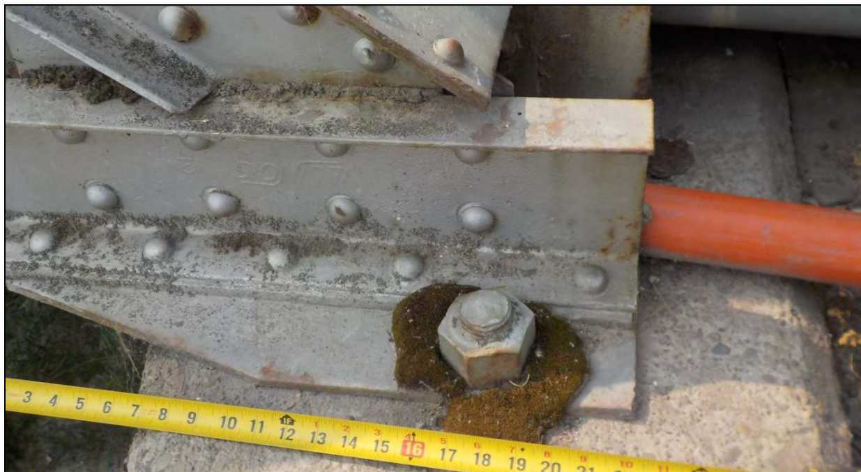
Photo 67: Bent 2, North Truss, Span 2 fixed bearing
