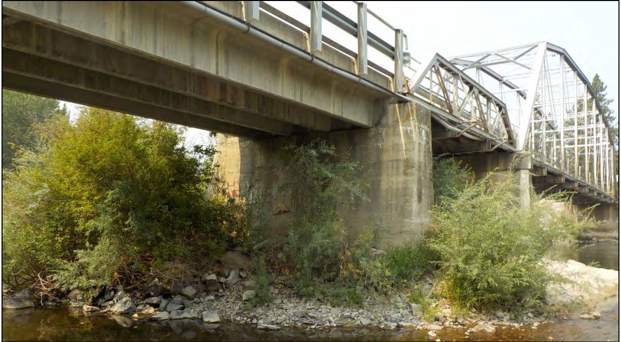
Photo 15: Bent 3 East Elevation looking west
