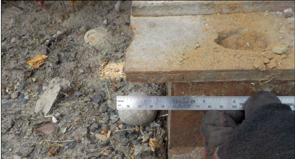
Photo 70: Bent 3, South Truss, Span 2 slider bearing
