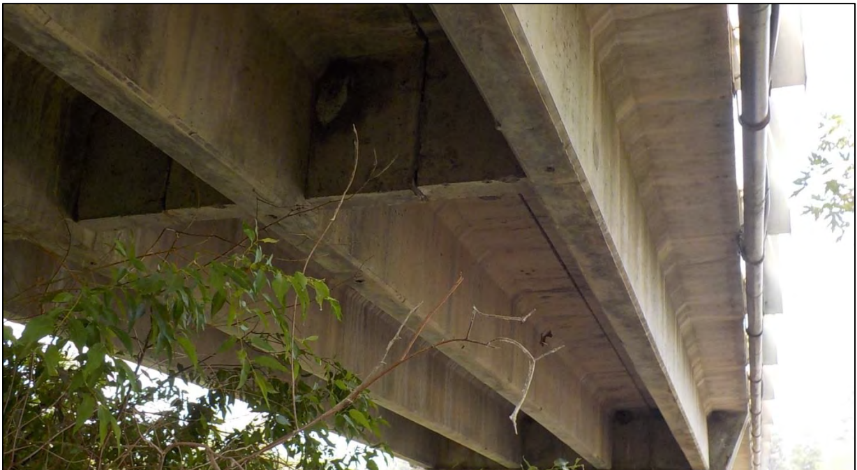
Photo 29: Typical underside of Span 3 deck
