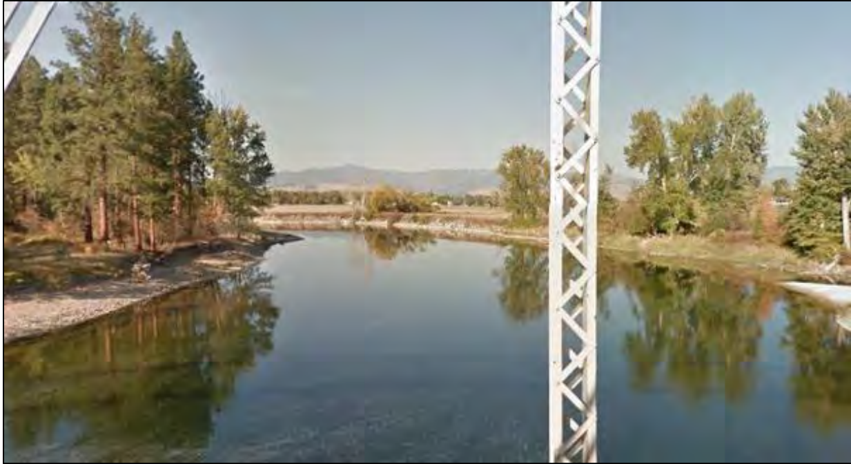
Photo 3: Looking downstream (north) at mid span
