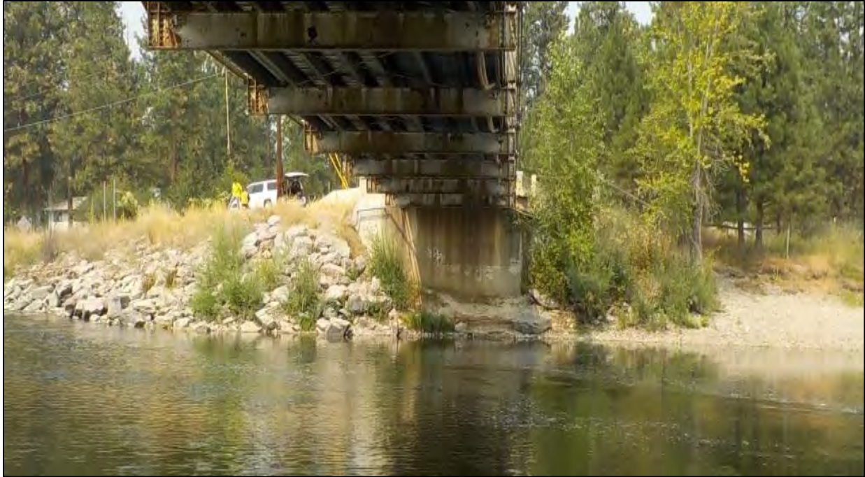
Photo 13: Abutment 1 East Elevation looking west
