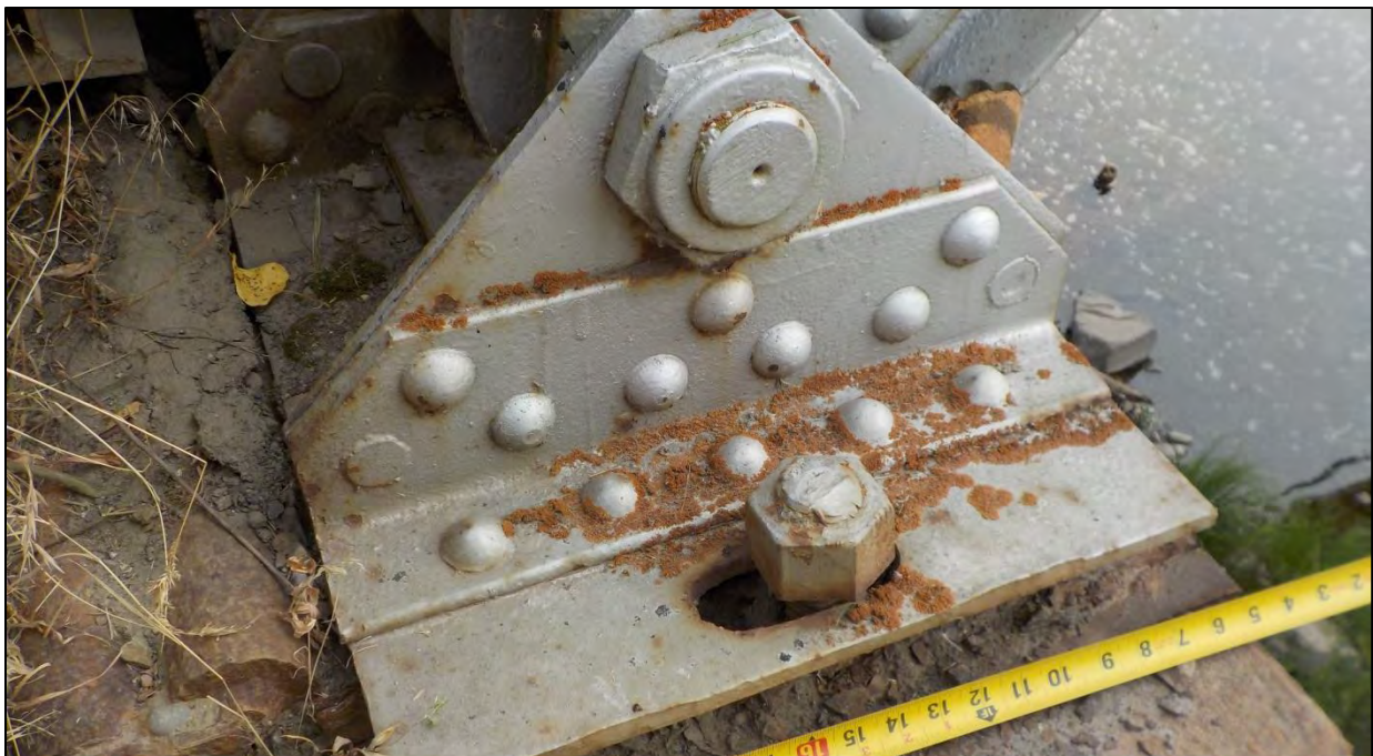
Photo 63: Abutment 1, South Truss roller bearing
