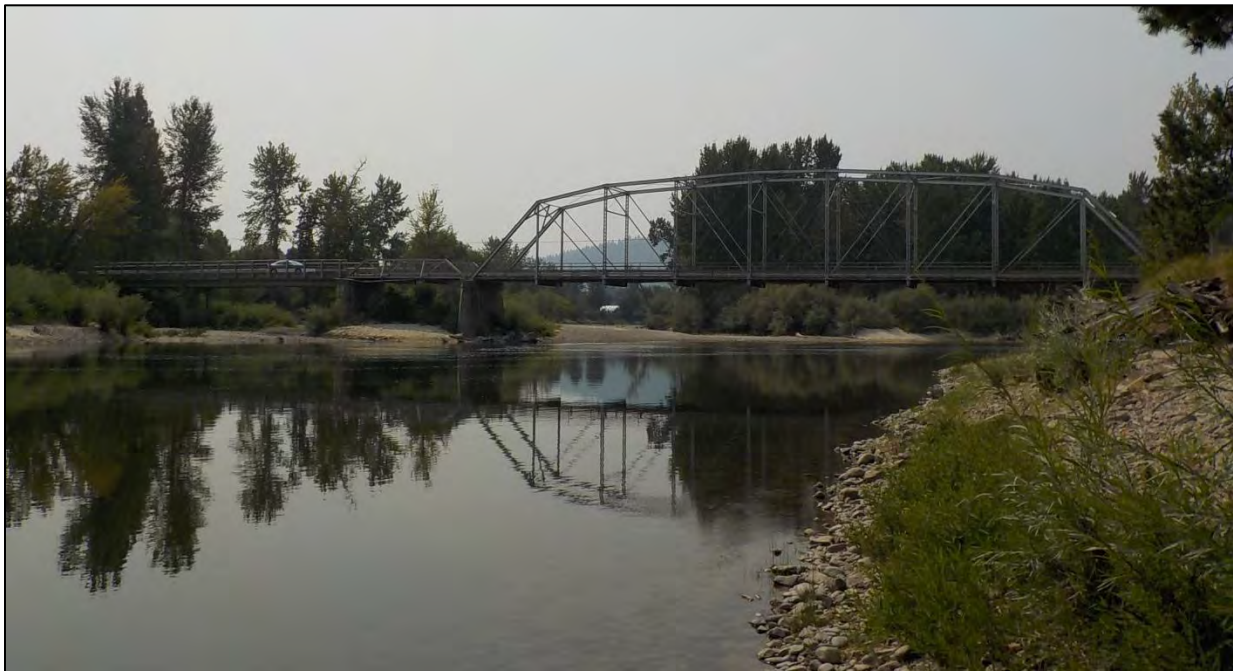
Photo 2: North Elevation looking south at bridge
