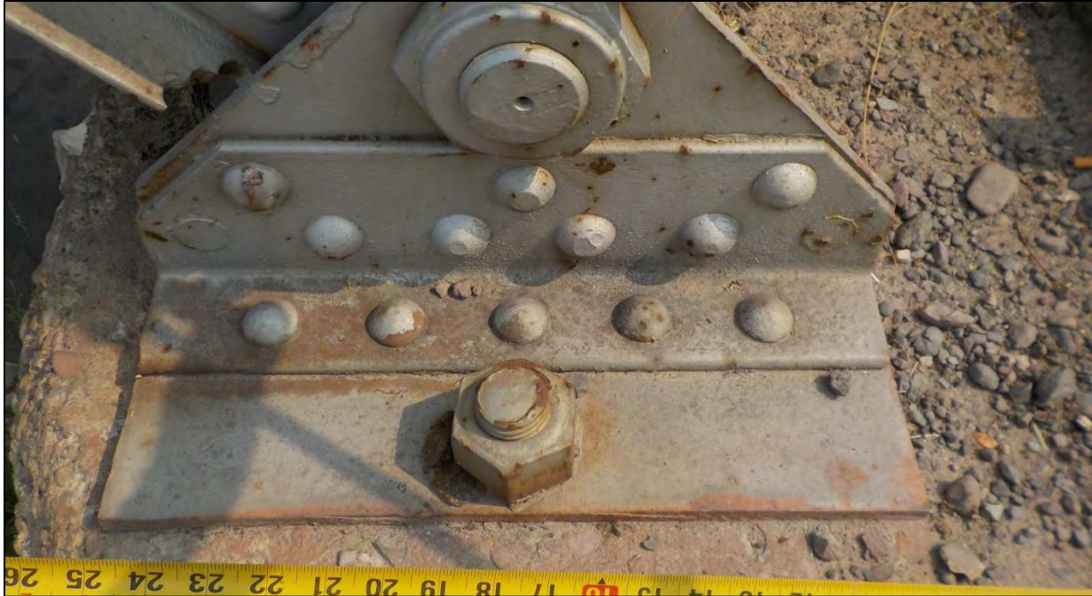
Photo 66: Bent 2, South Truss, Span 1 fixed bearing
