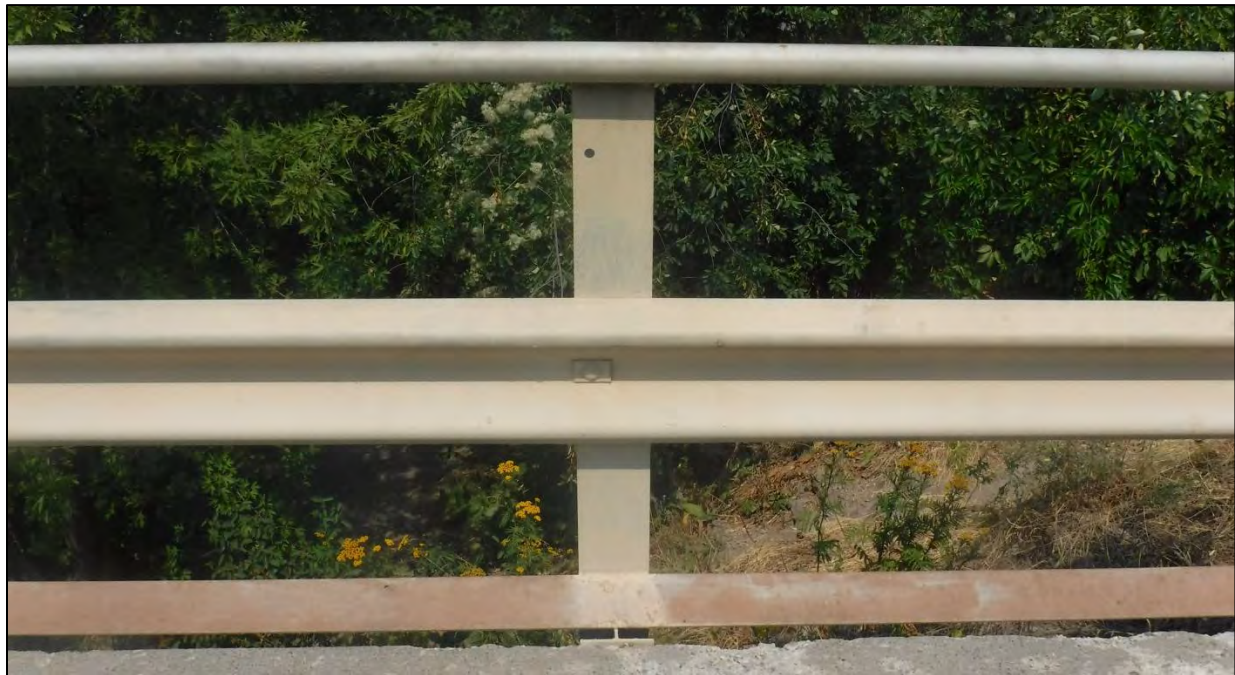
Photo 35: Bridge rail for Spans 3 and 4
