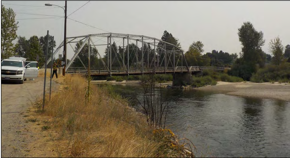
Photo 1: South Elevation looking north at bridge
