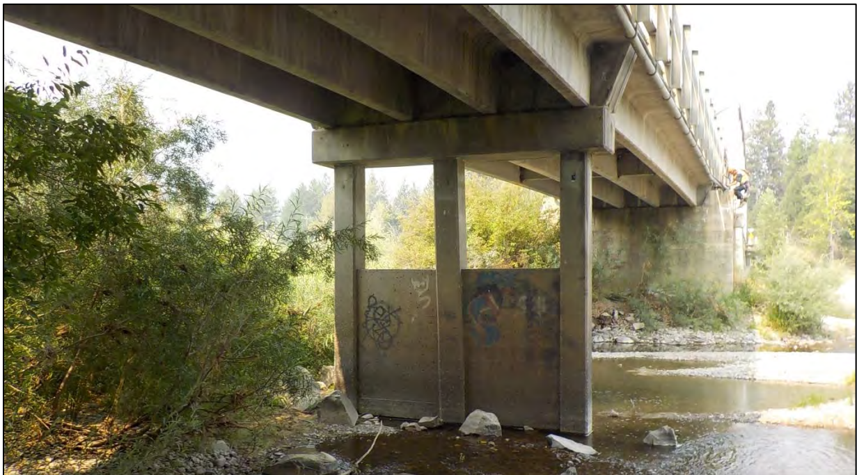
Photo 16: Bent 4 East Elevation looking west
