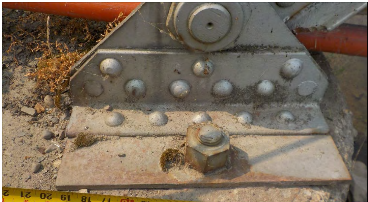
Photo 65: Bent 2, North Truss, Span 1 fixed bearing
