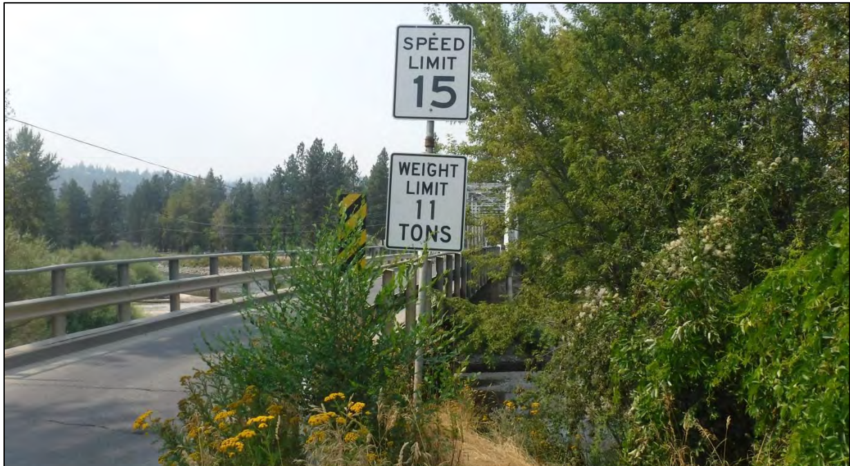
Photo 6: Weight Limit Sign on East End of bridge
