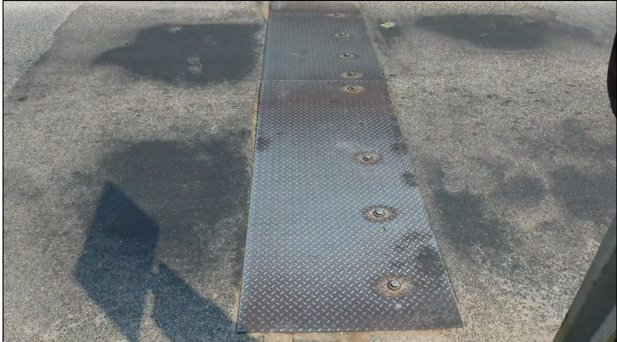
Photo 38: Joint 1 over Abutment 1 looking north at joint
