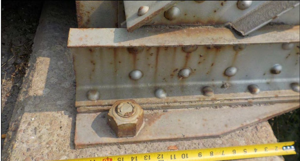
Photo 68: Bent 2, South Truss, Span 2 fixed bearing
