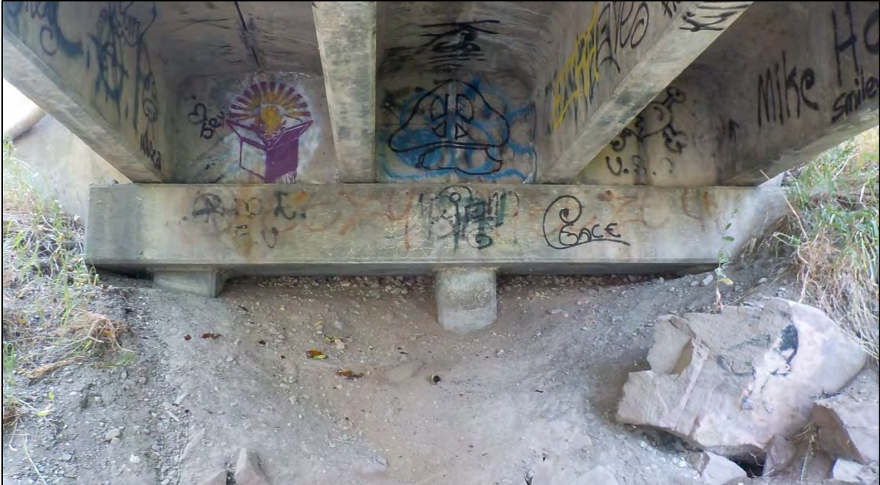
Photo 17: Abutment 5 West Elevation looking east
