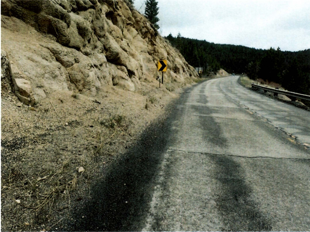
PHOTO 1: MT-2 (Harding Way/Pipestone Pass), facing southeast
