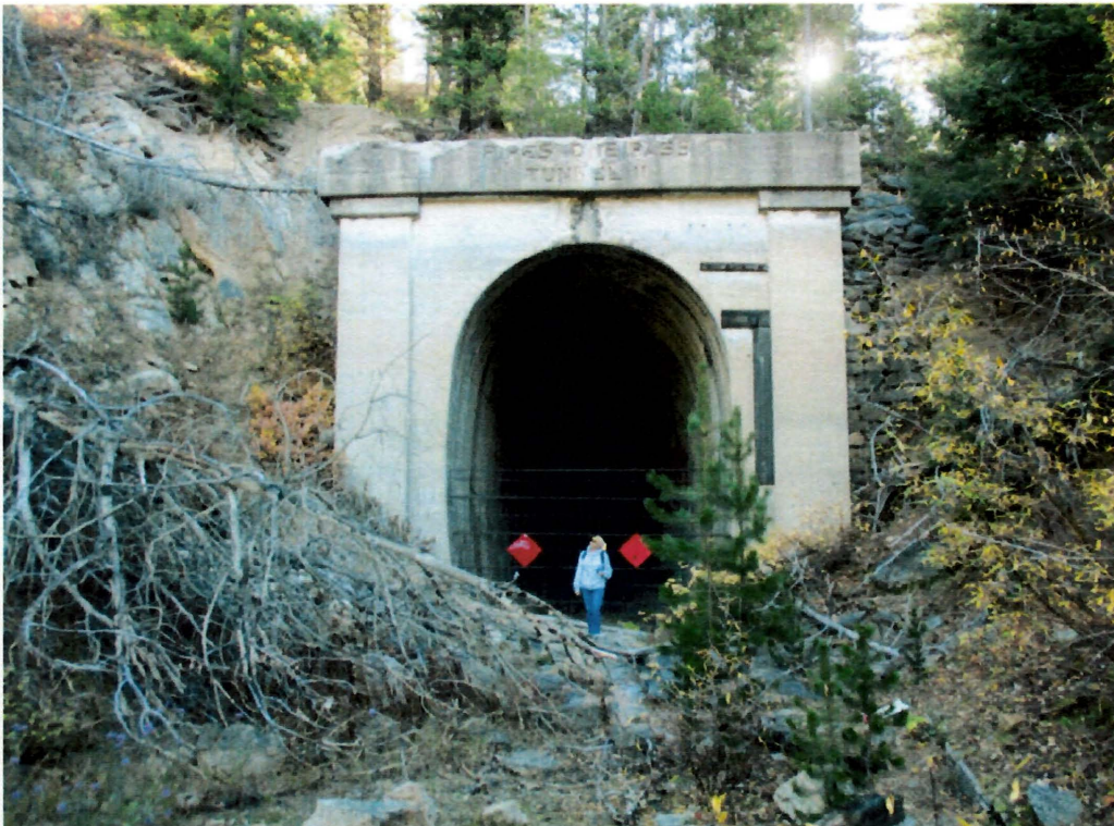
PHOTO 10: West end of Milwaukee Railroad Tunnel Number 11 (SB241162), facing southeast
