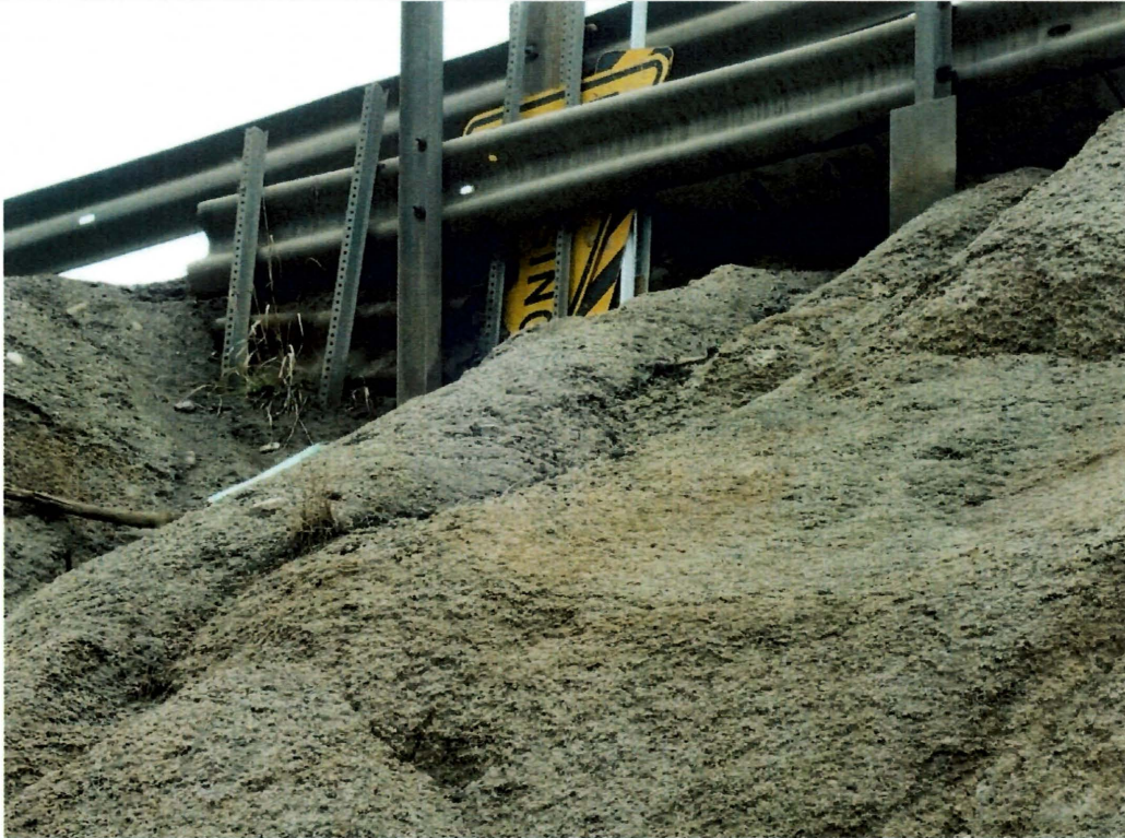
PHOTO 6: MT-2 (Harding Way/Pipestone Pass), facing northwest underneath roadway
