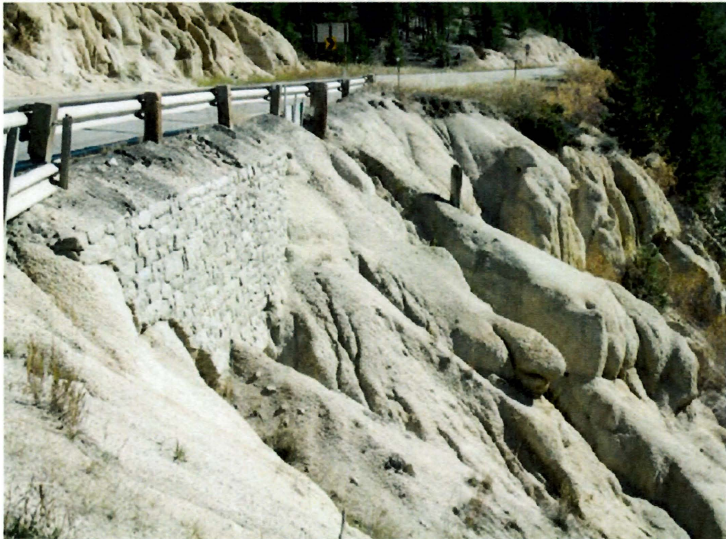
PHOTO 2: Harding Way Retaining Wall (24SB1163), facing southeast
