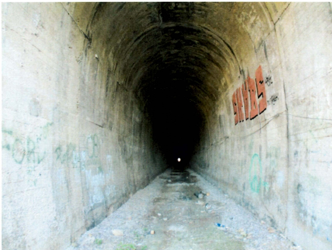
PHOTO 11: West interior of Milwaukee Railroad Tunnel Number 11 (SB241162), facing southeast
