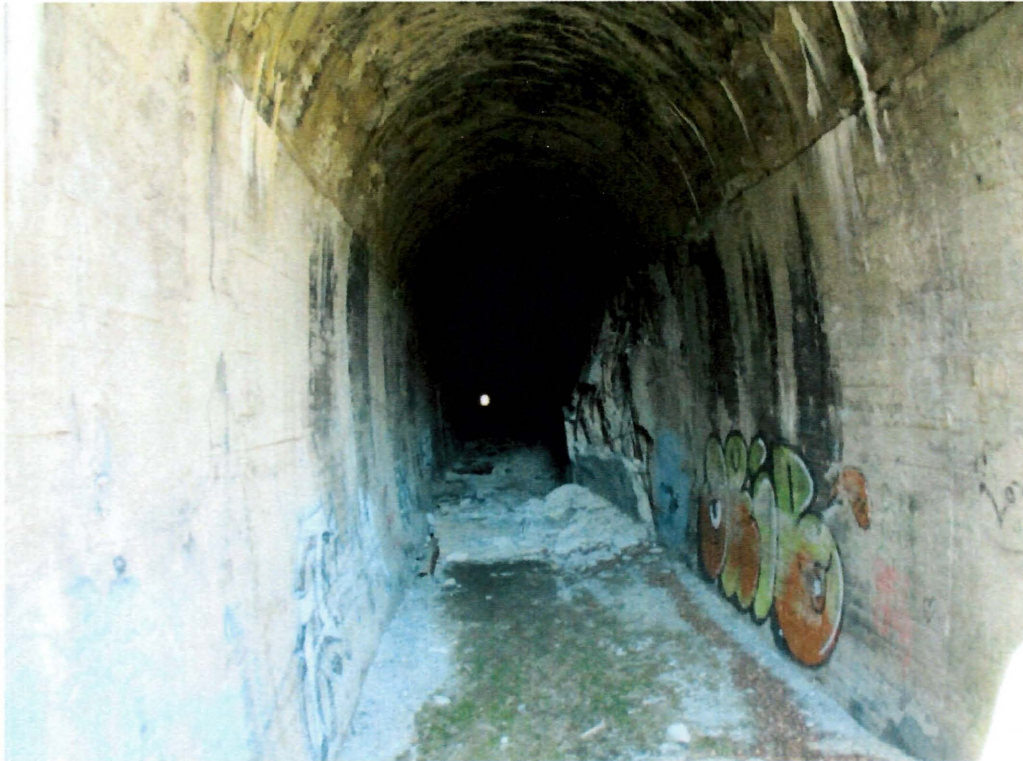
PHOTO 9: East interior of Milwaukee Railroad Tunnel Number 11 (SB241162), facing northwest
