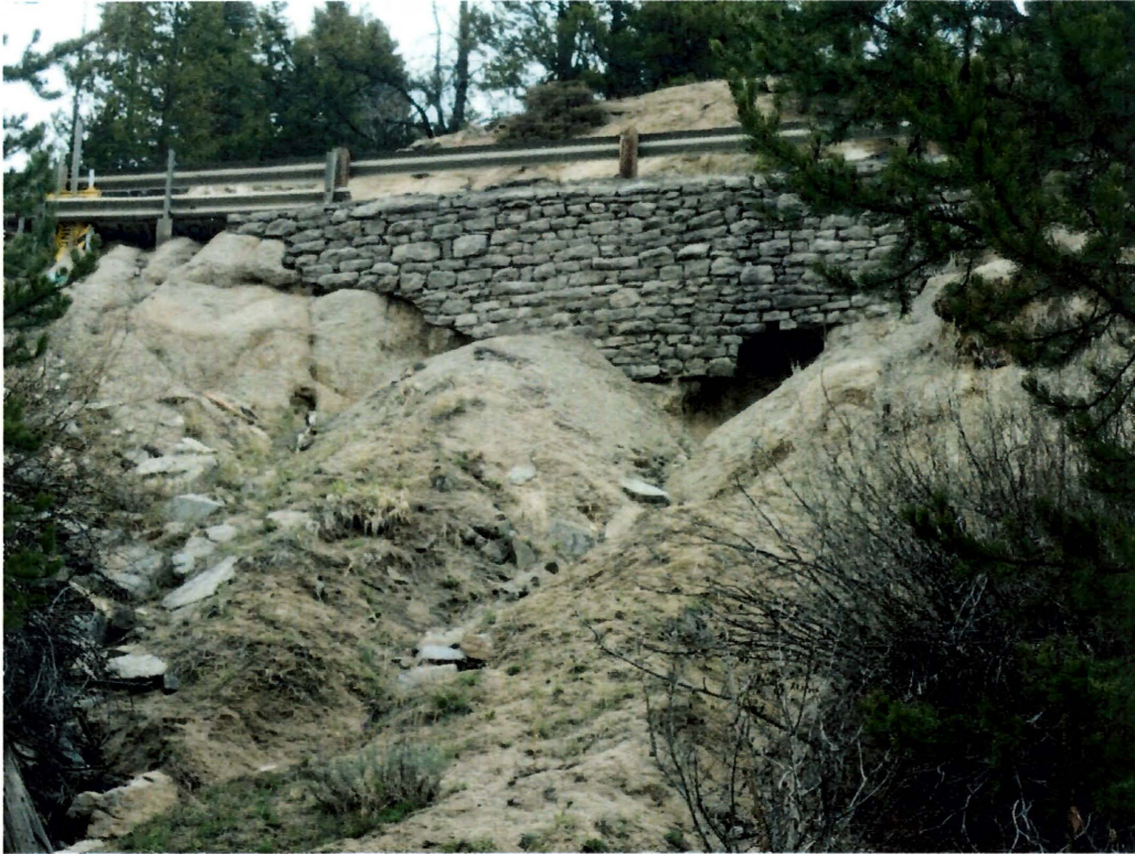
PHOTO 3: Harding Way Retaining Wall (24SB1163), facing north
