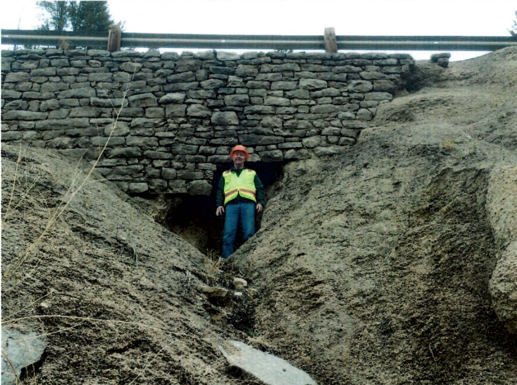
PHOTO 4: Harding Way Retaining Wall (24SB1163), facing north
