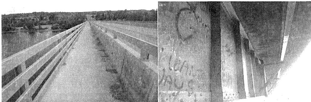
Cantilevered Path on the Yellowstone River
