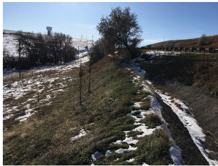
17. Photo Point 18 facing southwest showing concrete-lined ditch.
