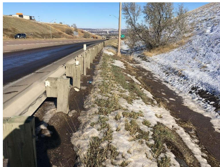
13. Photo Point 14 facing northeast showing Russian olive and concrete lined ditch
