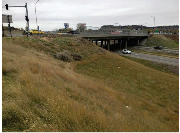
Photo 10: Johnson Interchange area and I-90, looking northwest.
