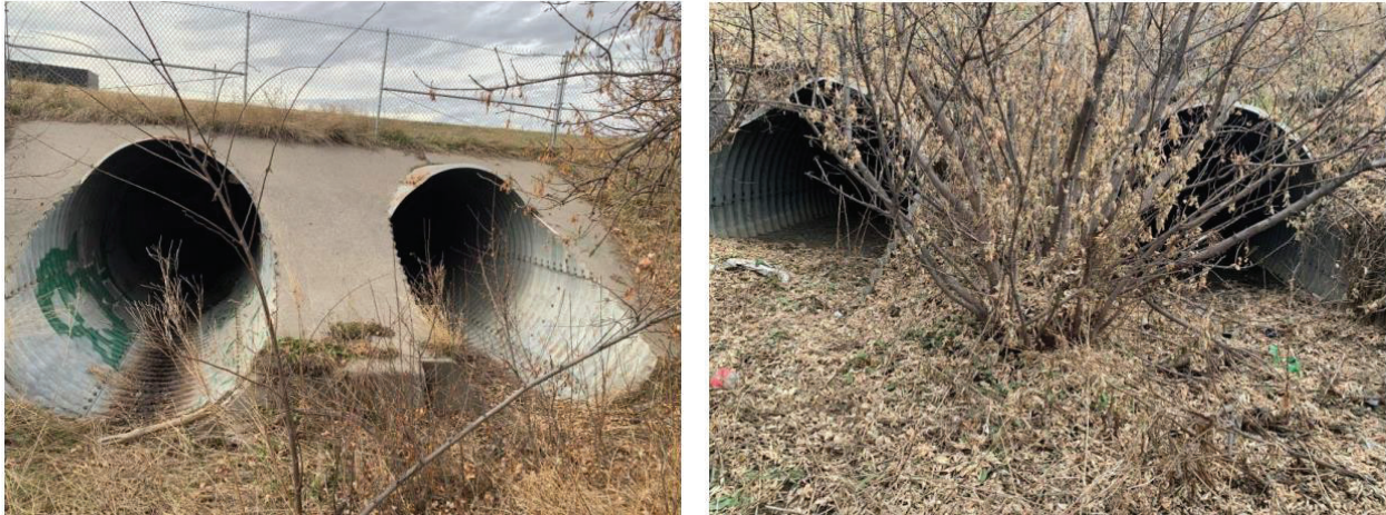
Figure 3-4. Dry Creek, Dual 96-in. CSP Entrance and Exit
