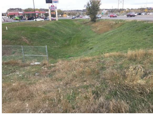
Photo 8: Swales on NW side of Lockwood Interchange
