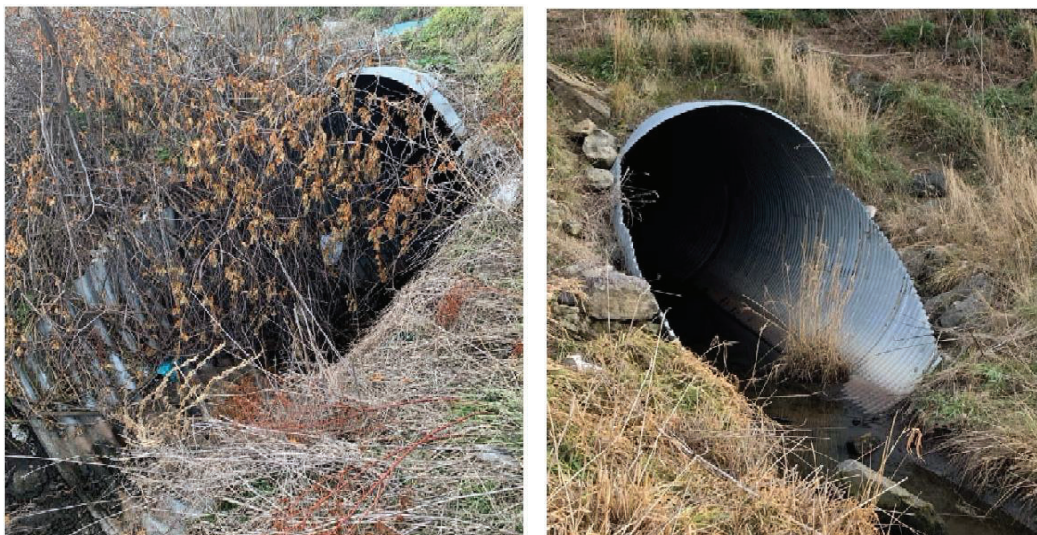
Figure 3-5. Unnamed Tributary, 84-in. CSP Entrance and Exit,
