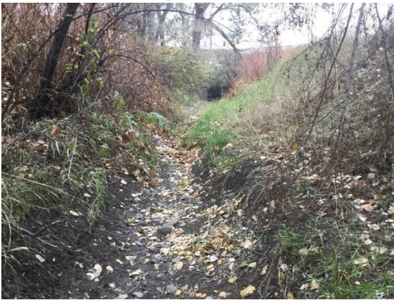
Photo 3: Lockwood Irrigation ditch
