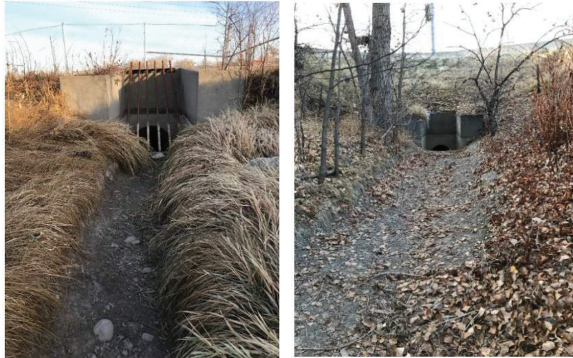
Figure 3-2. Lockwood Irrigation District 60-ft. Lift Ditch, 48-in. RCP Siphon Entrance and Exit
