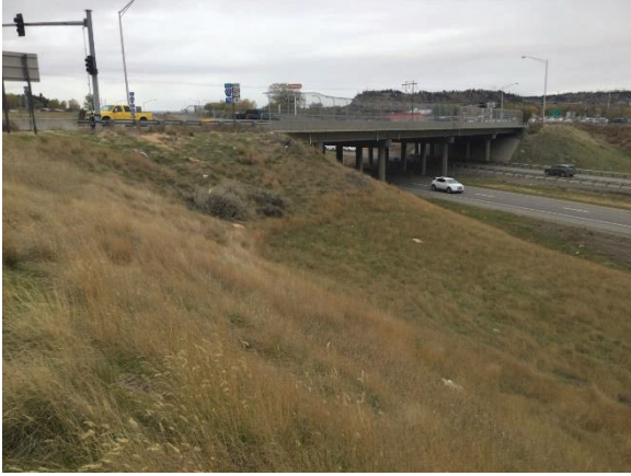
Photo 7: I-90 and Old US-87 overpass
