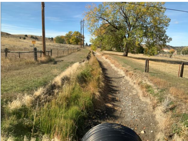
Photo 5: Upper Lift Ditch at Coburn Road (west side of road), looking west.
