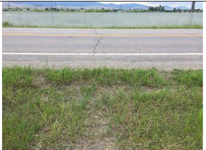
**PHOTOGRAPH 48** Crack in asphalt over top of culvert C11, RP 10.2.
