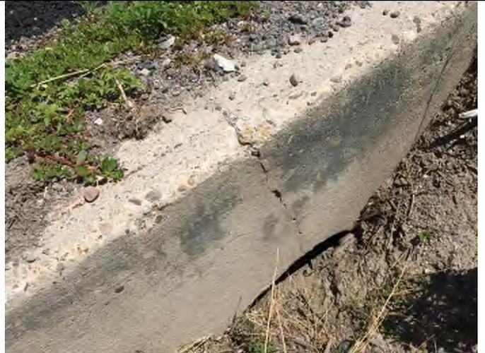
**PHOTOGRAPH 16** Crack in concrete at C4 outlet, RP 7.8.
