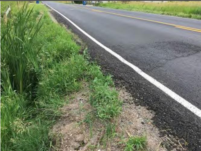
**PHOTOGRAPH 35** Pavement depression over culvert C8 outlet, RP 9.1.
