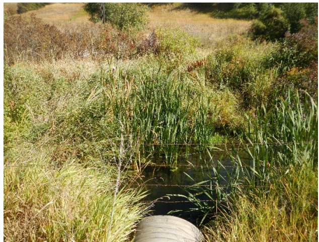
Photo 12: LaValle Creek culvert crossing at approximately RP 8.4, looking east.
