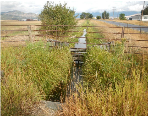
Photo 9: Irrigation ditch at approximately RP 8.8, near Fairbanks Lane, looking north.
