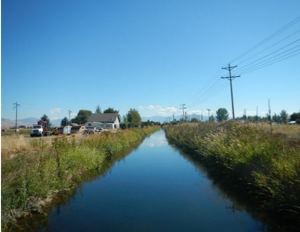
Photo 13: Frenchtown Irrigation District Ditch at approximately RP 7.7, looking south.
