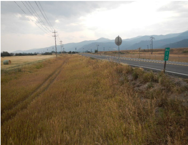
Photo 3: Roadside ditch, RP 10, looking south.
