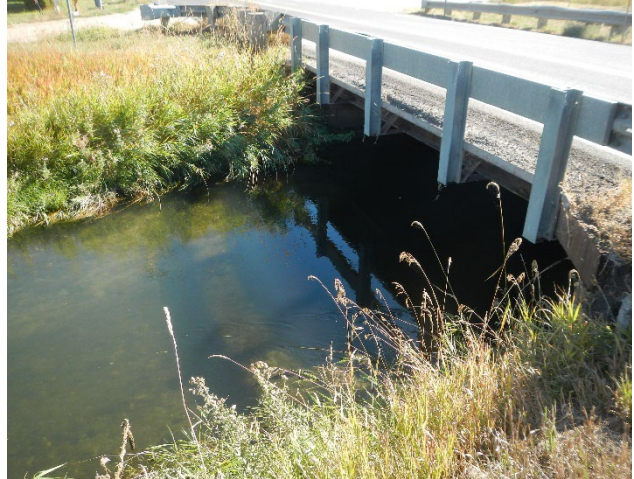
Photo 14: Bridge structure located at RP 7.3 spanning the Frenchtown Irrigation District Ditch
