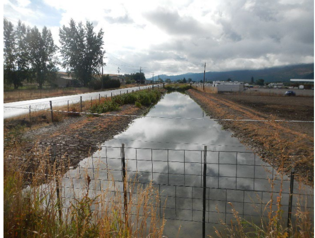
Photo 8: Irrigation ditch at approximately RP 8.8, near Fairbanks Lane, looking south.
