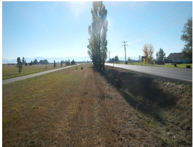
Photo 16: Shared-use path (left) and Mullan Road (right) at approximately RP 6.6.
