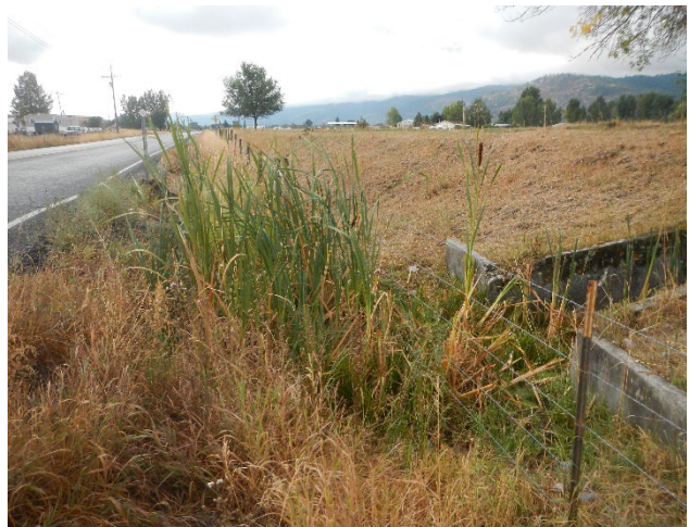
Photo 10: Irrigation drainage crossing structure and ditch wetlands at approximately RP 9.1, looking south
