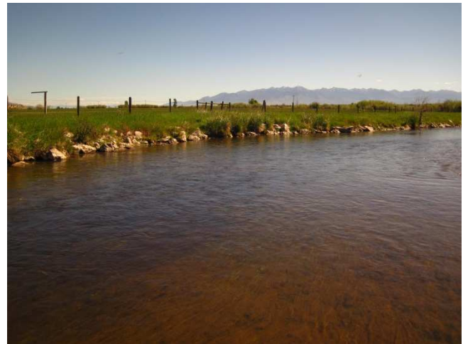
Photo 16 Desc: Riprap along left bank of Beaverhead River.
