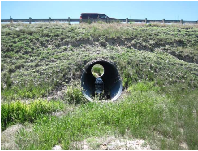
Photo 7 Desc: Unnamed spring creek culvert beneath Hwy 41.
