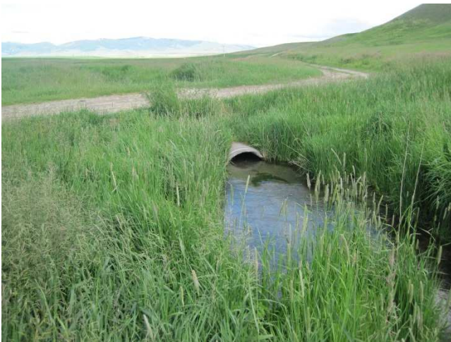
Photo 5 Desc: Culvert on Stone Creek upstream of Hwy 41.
