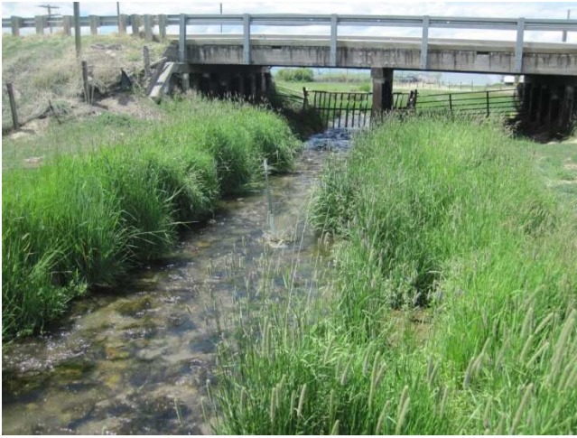
Photo 1 Desc: Stone Creek crossing at Highway 41.
