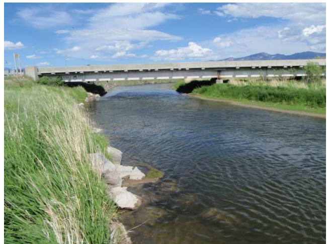
Photo 12 Desc: Hwy 41 bridge over Beaverhead River.
