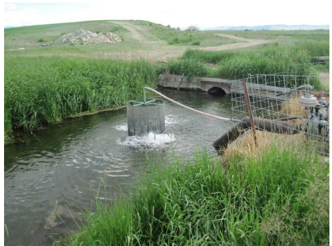
Photo 6 Desc: Check structure, pump, and culvert on Stone Creek.
