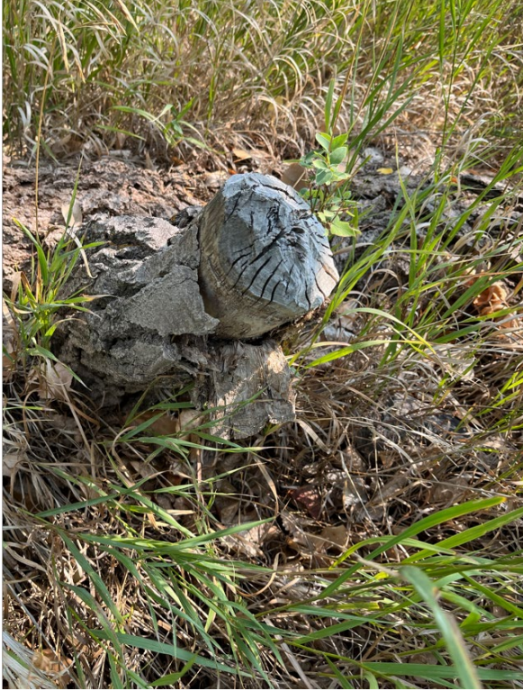
Photo 5: Old beaver sign near the east bridge abutment.
