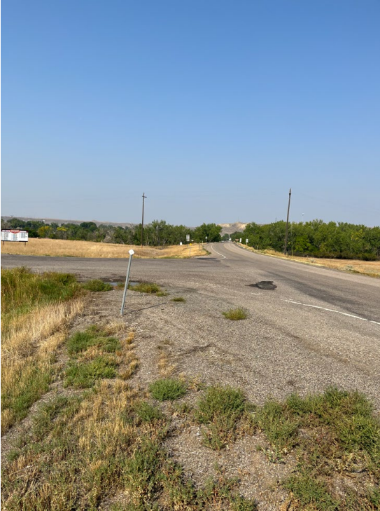
Photo 1: Junction of MT-80 and S-228, looking northwest towards MT-80 bridge.
