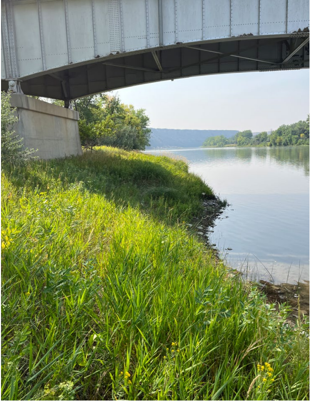
Photo 9: East bank MT-80 bridge, looking upstream.
