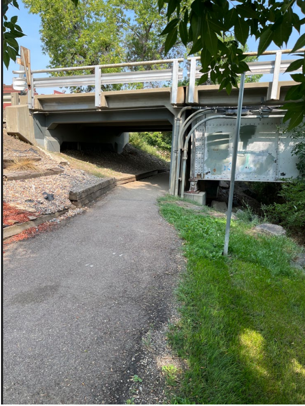
Photo 13: Levee trail system passing under west bridge abutment
