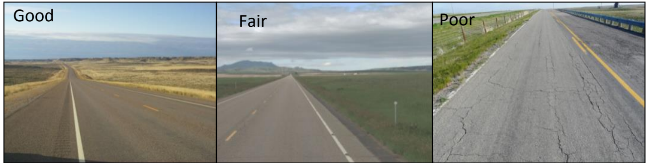
Figure 35: Montana Pavement Condition
