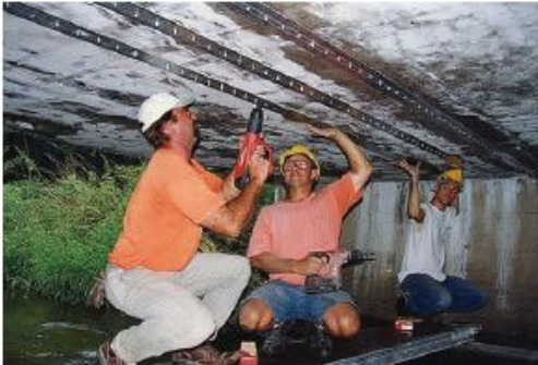
Workers installed SAFSTRIP® on this bridge in Edgerton, Wisconsin, using the MF-FRP system. The load rating for the bridge increased from HS-17 to HS-25 as a result.
