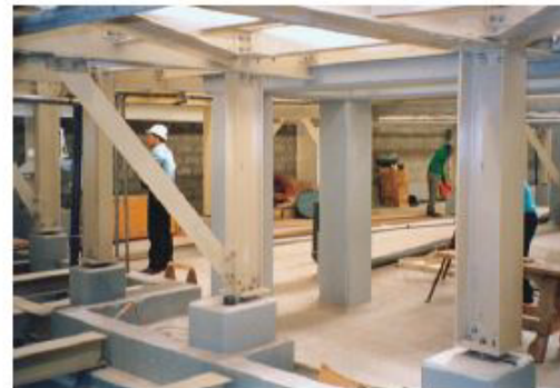
EXTREN® structural shapes were used in a SKEW copper refinery because of the highly corrosive environment.
