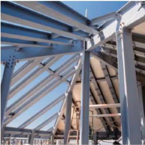
This entire rooftop structure was built using EXTREN®, to take advantage of its transparency to RF and cellular signals.
