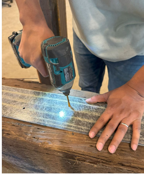
Figure 30: Attaching strip to the beam
