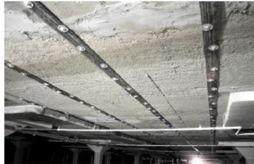
This underground parking garage for an apartment complex in Ontario, Canada, recently underwent a concrete support renovation. To provide the necessary improvements, SAFSTRIP® was installed with a small team and minimal onsite equipment.
