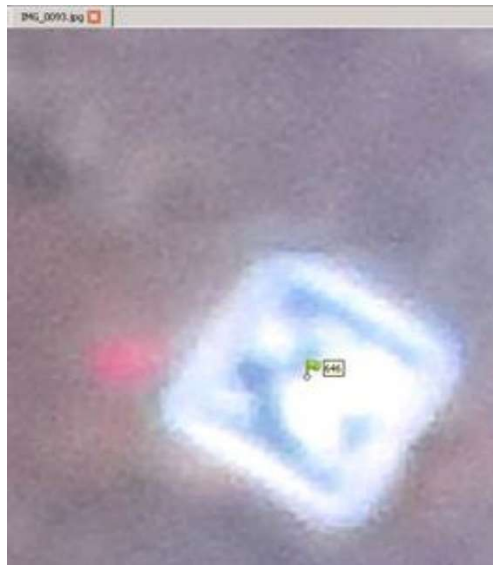
Example of poor image quality over a control panel
