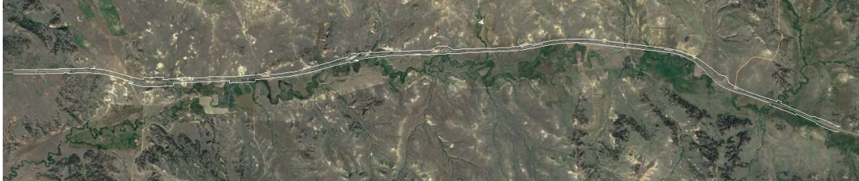
Overview of Ashland Corridor
