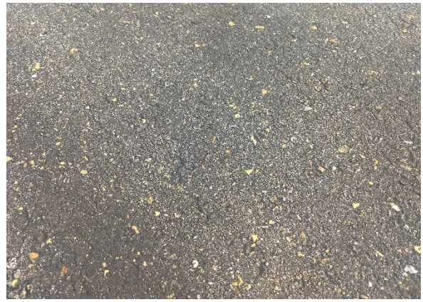
T-3, Surface with Weathering
