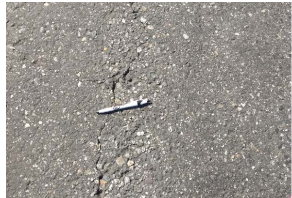
A-2, Cracking
