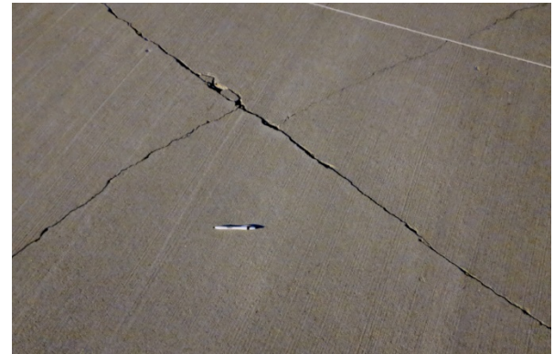
A-6, Shattered Slab
