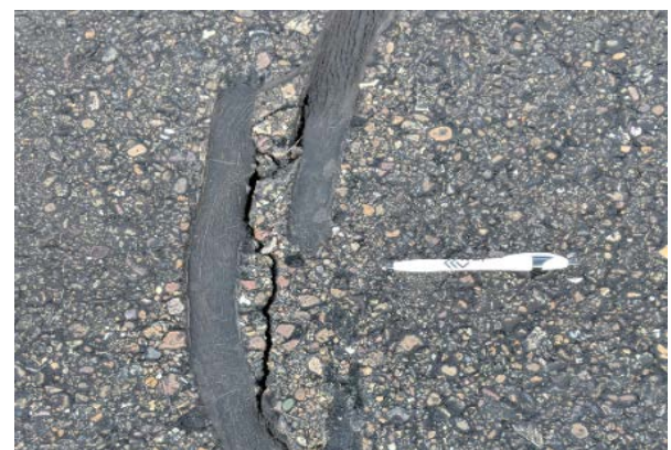
T-11, Cracking
