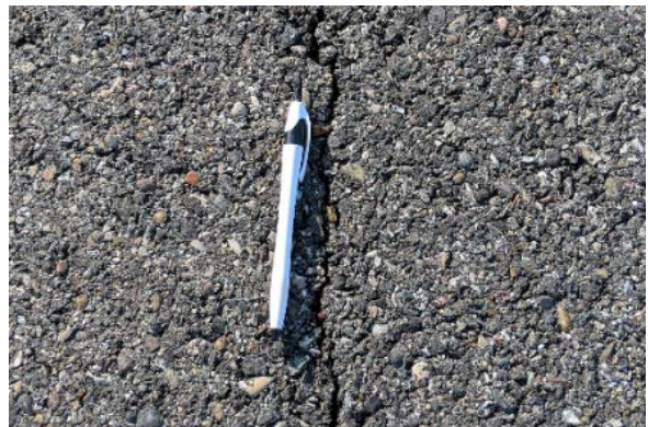
R-1, Cracking
