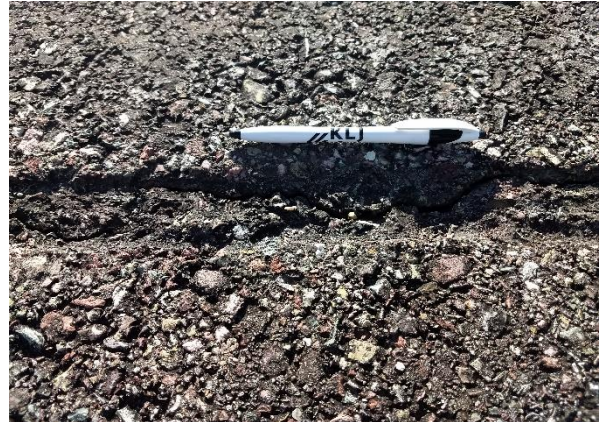
A-1, Routed Crack with Sealant
