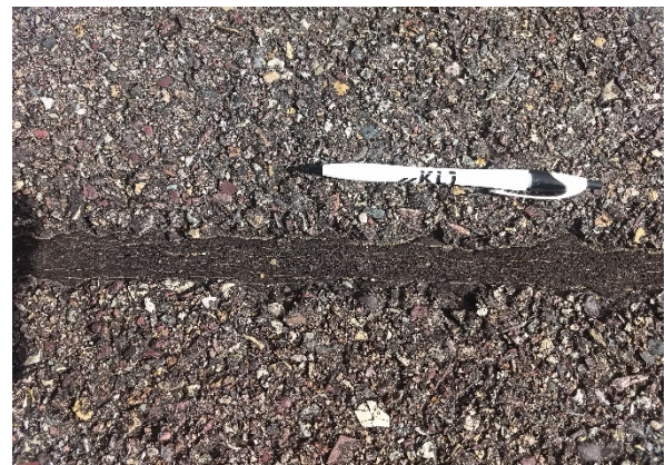
R-11, Sealed Crack
