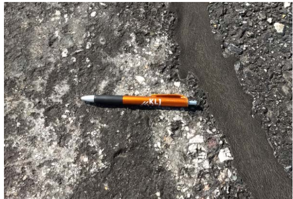
A-11, Cracking
