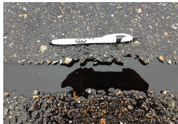
R-1, Sealed Crack
