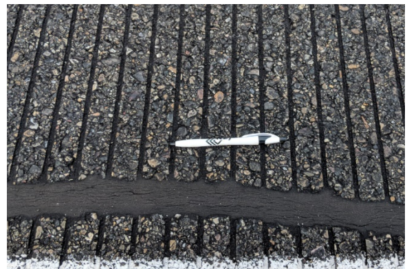
R-1, Crack-Sealed
