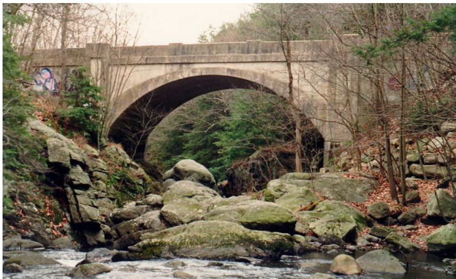
Figure 5.7.5-1 A Closed Spandrel Reinforced Concrete Arch Bridge
