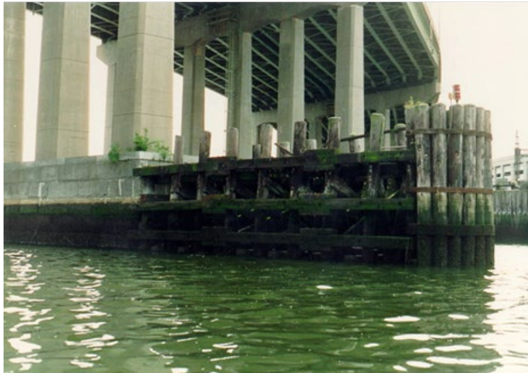
Figure 5.9.1-1 Timber Fender System with Navigation Lights.
