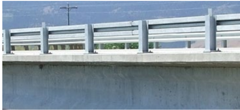
Figure 3.5.1-1 T-101 Rail on Concrete Deck: Code 1
