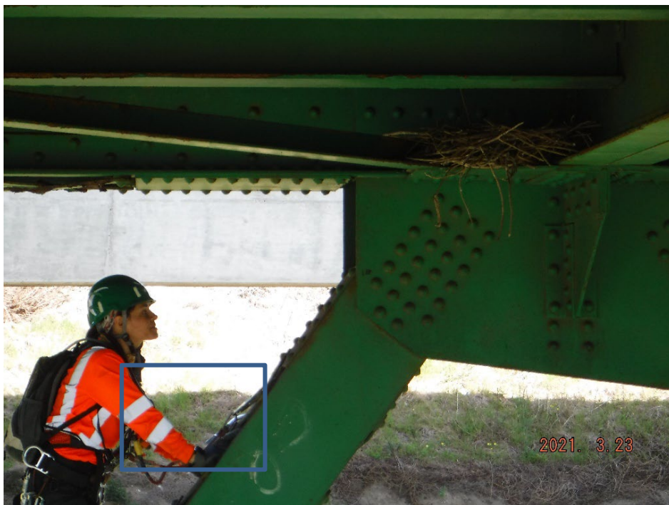
Figure 4.4.2-2 Bridge Inspector Using Climbing Techniques (Level B Climbing)
