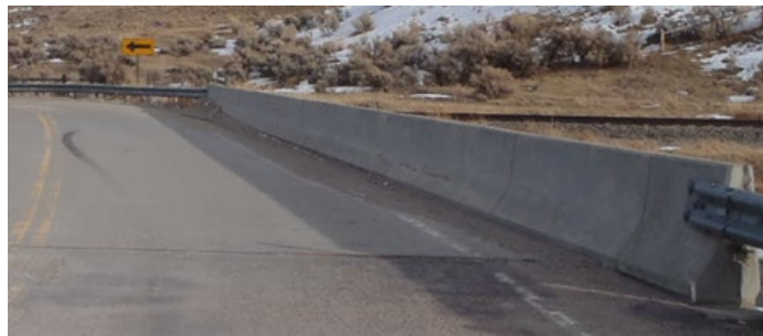
Figure 3.5.1-2 Concrete Barrier Rail: Code 1
