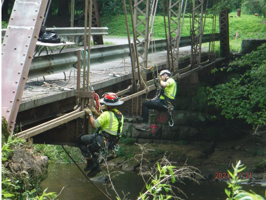
Figure 4.4.2-3 Bridge Inspectors using Rope Access Techniques (Level C Climbing)
