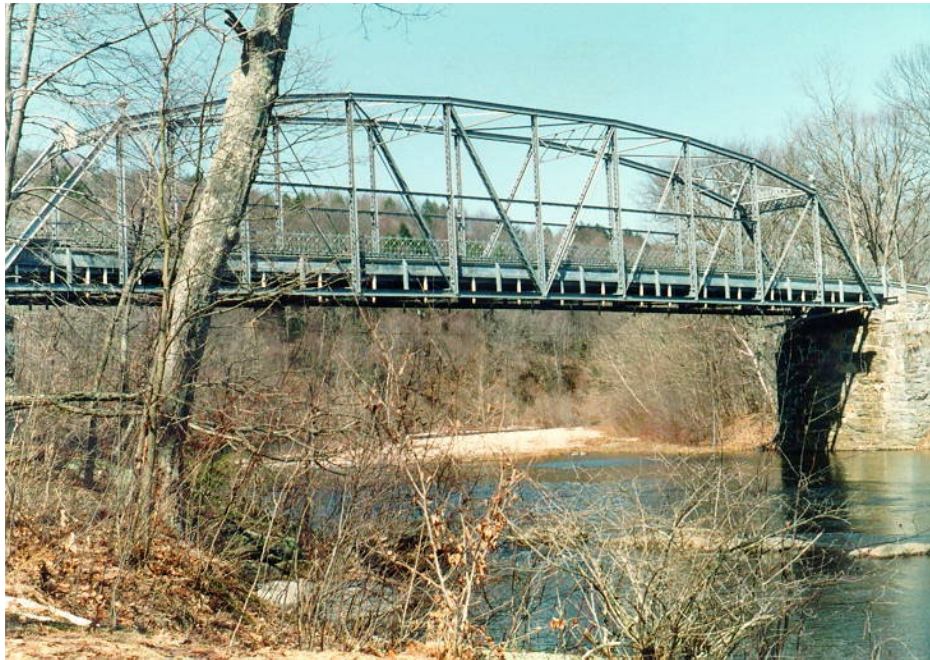
Figure 5.7.11-1 Historic Steel Through Truss Bridge.
