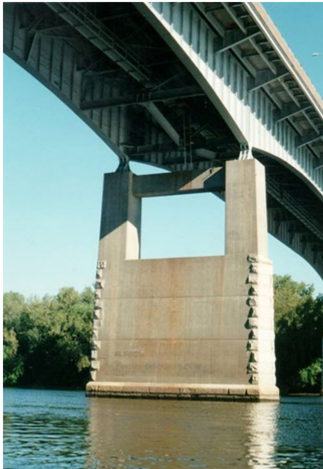
Figure 5.8.1-2 Tall Concrete Pier with Decorative Stone Masonry Facing
