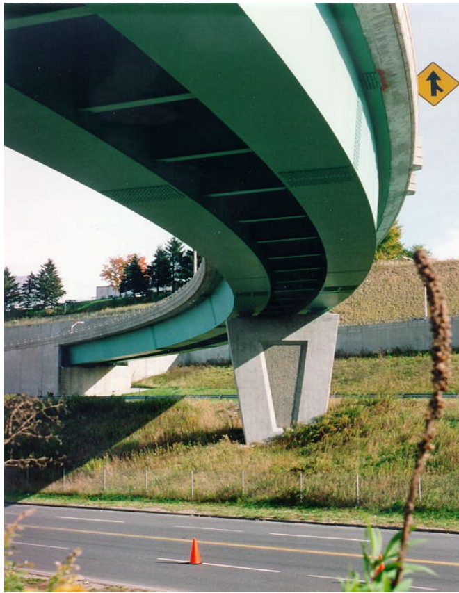
Figure 5.7.10-1 Curved Steel Box Girder Bridge.
