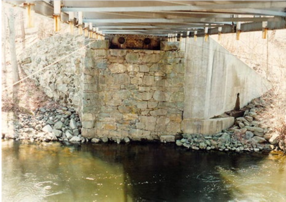
Figure 5.8.2-1 Tall Stone Masonry Bridge Abutment with Newer Concrete Wingwall Added.
