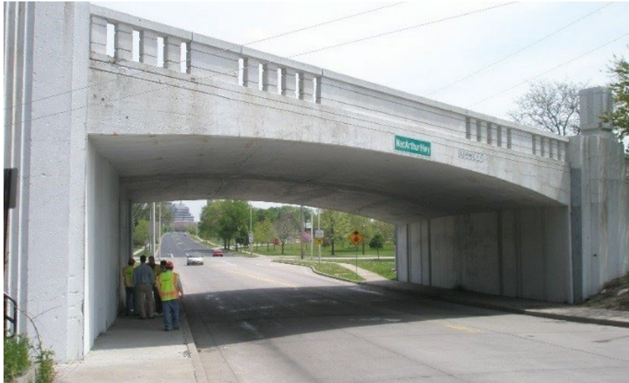
Figure 5.7.5-2 Single-span Rectangular Concrete Rigid Frame Bridge
