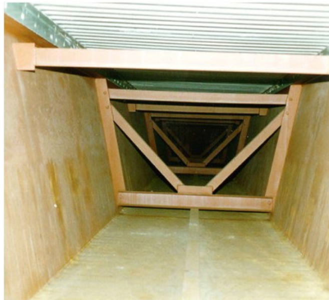
Figure 5.7.10-2 Inside Steel Box Girder.
