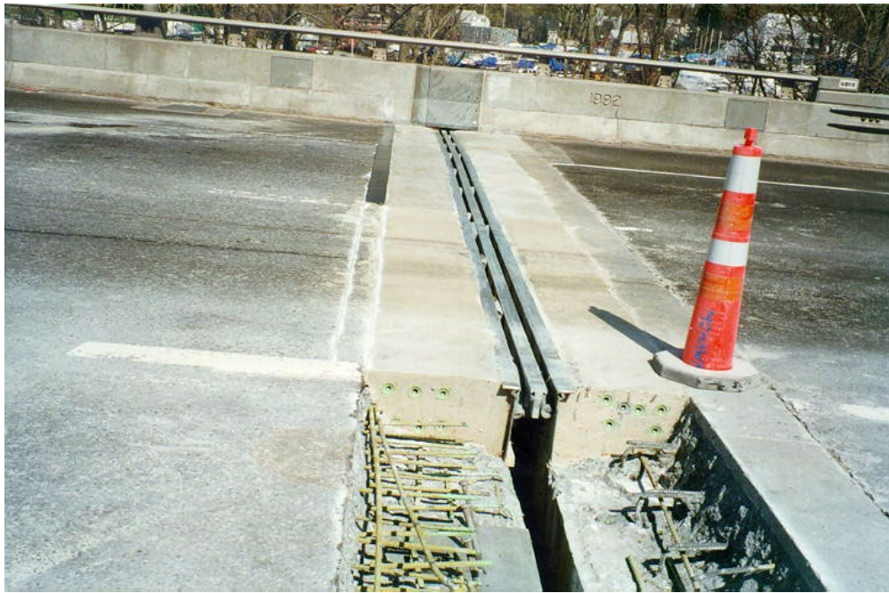
Figure 5.6.10-3 Modular Type Expansion Joint Replacement.
