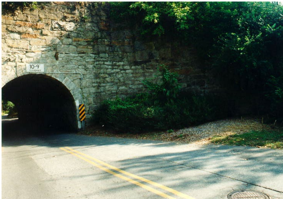
Figure 5.7.13-1 Stone Masonry Arch and Spandrel Wall
