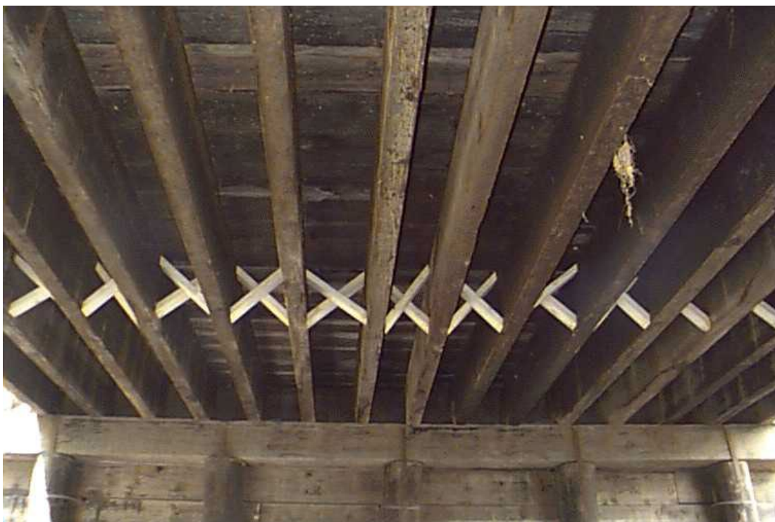
Figure 5.7.12-2 Underside View of a Solid Sawn Multi-Beam Timber Bridge.
