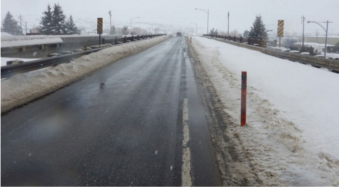
Figure 4.1.8-1 A follow-up inspection is required to check the condition of the bridge deck and associated elements (joints, rail, etc.).
