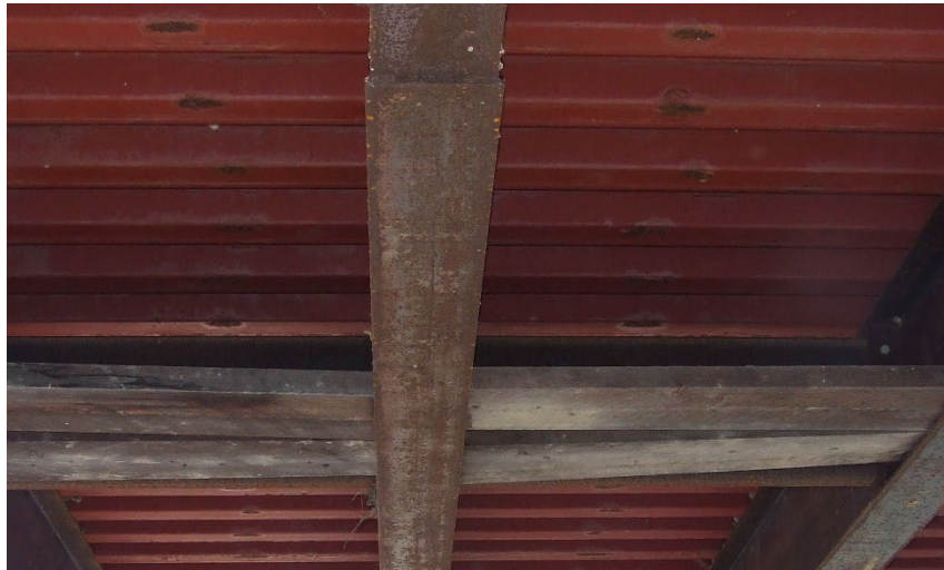
Figure 5.6.3-1 Underside of Corrugated Metal Deck
