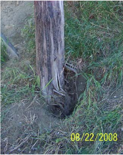
Failed timber pile due to decay
