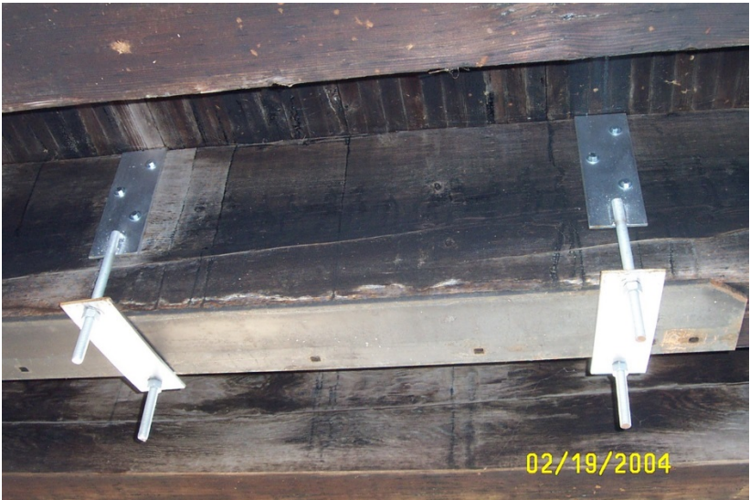
Steel hanger girder repair with multiple bolts
