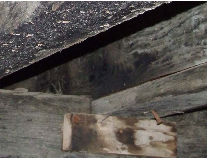
Split propagating from a notch
