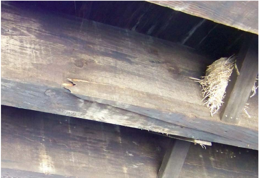
Moderate Crack
