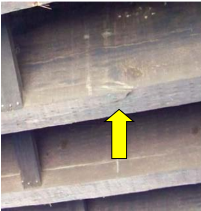
Minor Crack (both photos are of same crack)
