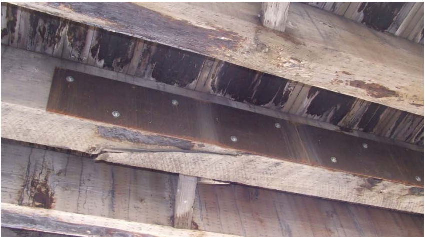
Steel plate girder repair
