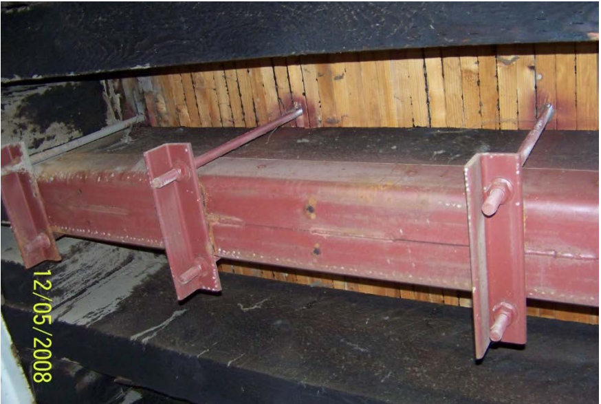
Steel hanger girder repair – through deck hangers with bottom plates
