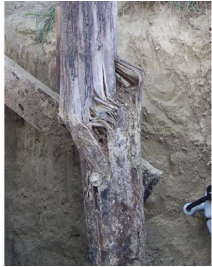
Failed timber pile due to decay
