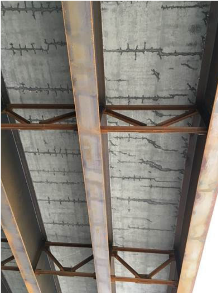
Northbound Structure built 2016
