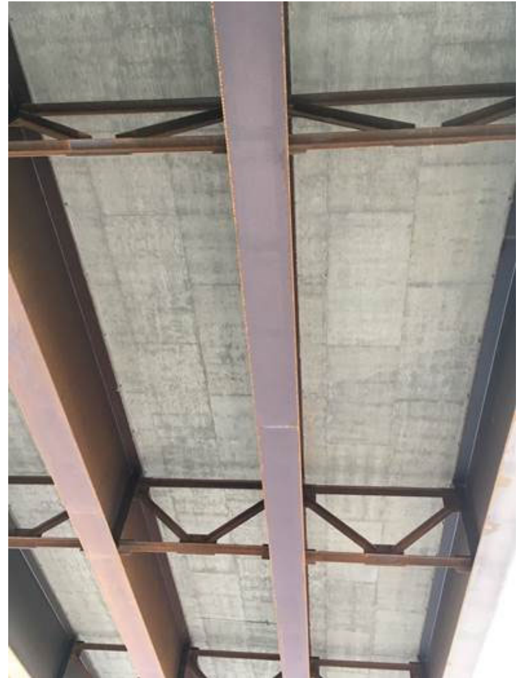
Southbound Structure built 2017
