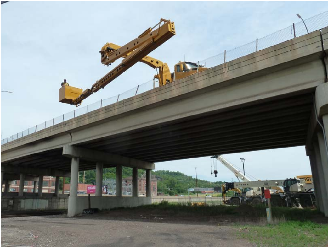
OPEN BOOM-2 AND BOOM-3
